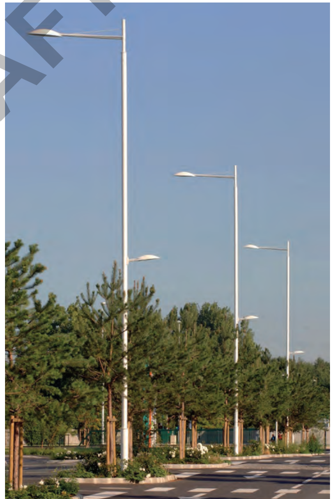
Roadway and Pedestrian Scale Lighting
