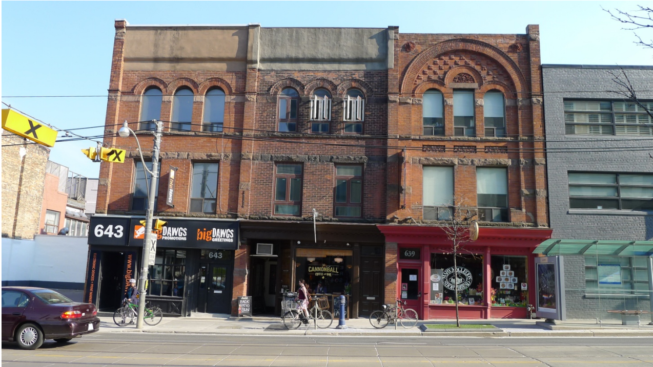
19. Smith Block, 639-643 Queen St. E.: showing the north elevations of the remaining three blocks at the west end of the original block. (HPS)
