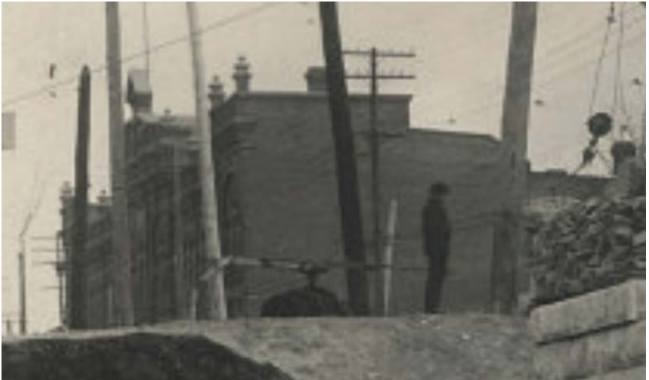
13. Detail of "East Abutment, Queen Street Bridge over the Don, December 4, 1899" : showing the Smith Block. Note the central 'broken' pediment with the higher pediment emerging at above. The side wall is blank perhaps in anticipation of future development on the block. (CTA, Fonds 200, Series 376, Item 37)
