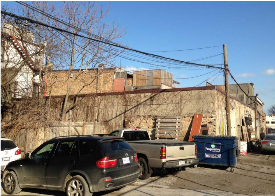
21. Smith Block, 643-649 Queen St. E.: showing the rear, south, elevation of 643 Queen St. E. and the single storey warehouse block. N.B. These rear elevations and additions are not identified as heritage attributes. (HPS)
