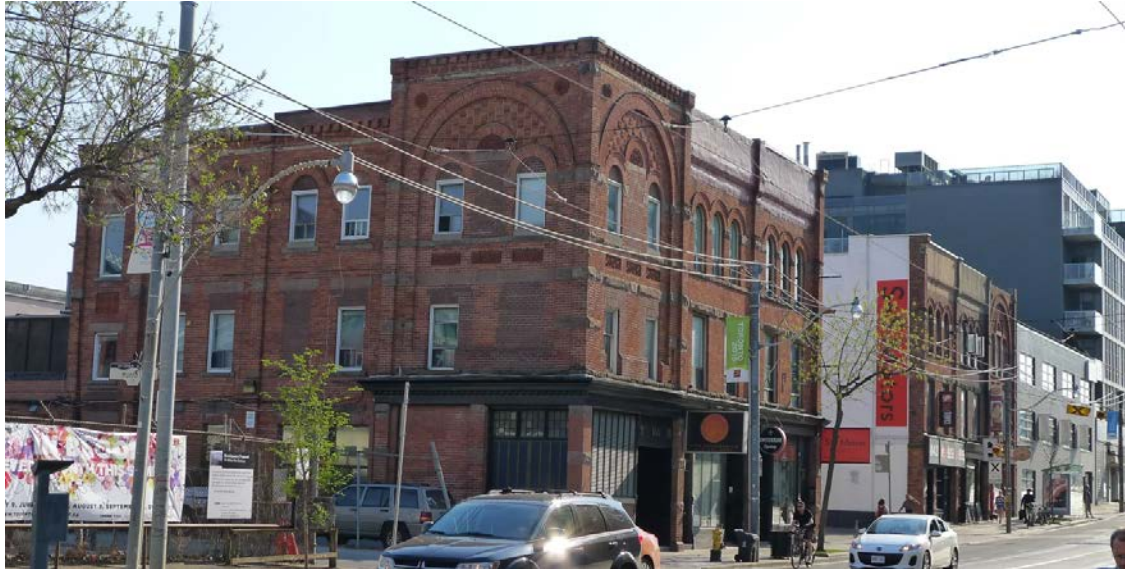
Smith Block, 651-655 Queen Street East and 643-639 Queen Street East : showing the remaining sections of the Smith Block on the south side of Queen Street East ( Heritage Preservation Services, 2015 [HPS] )
