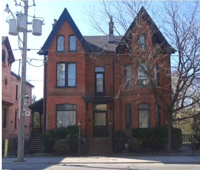
201 and 203 Gerrard Street East
