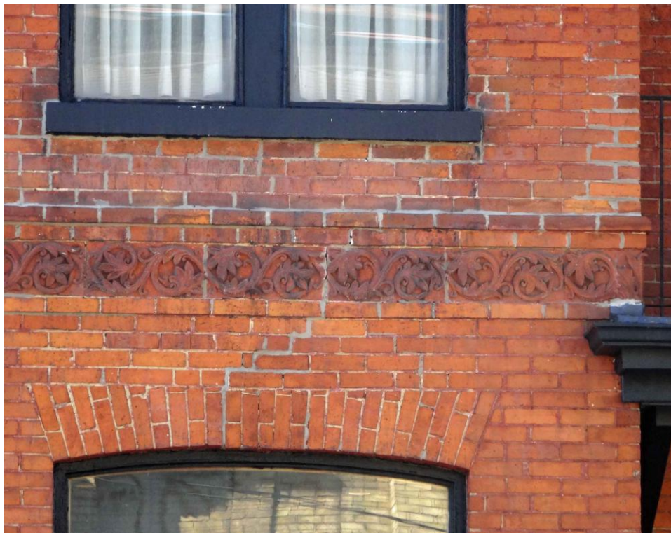
12. Current Photograph, 201 and 203 Gerrard Street East, 2016 : showing the rear (south) walls (above), and the detailing on the principal (north) elevations with the decorative terra cotta (below) (Heritage Preservation Services, 2016).
