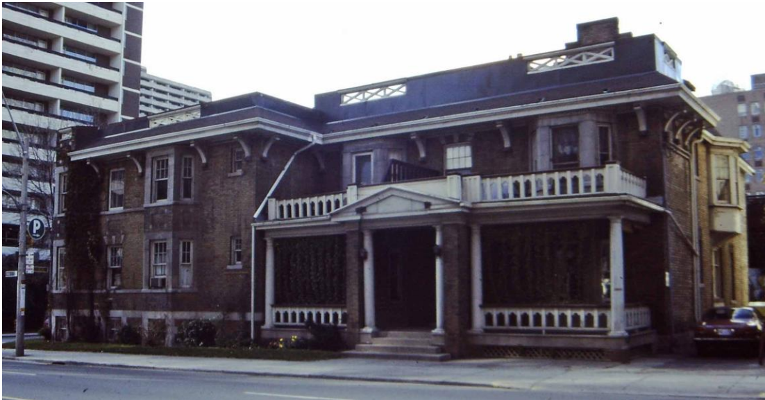
13. Archival Photograph, 628 Church Street, 1990 : this view of the east elevation of the Manhattan Apartments on Church Street shows the surviving late 19th century house form building incorporated in the complex on the right (Toronto Historical Board).
