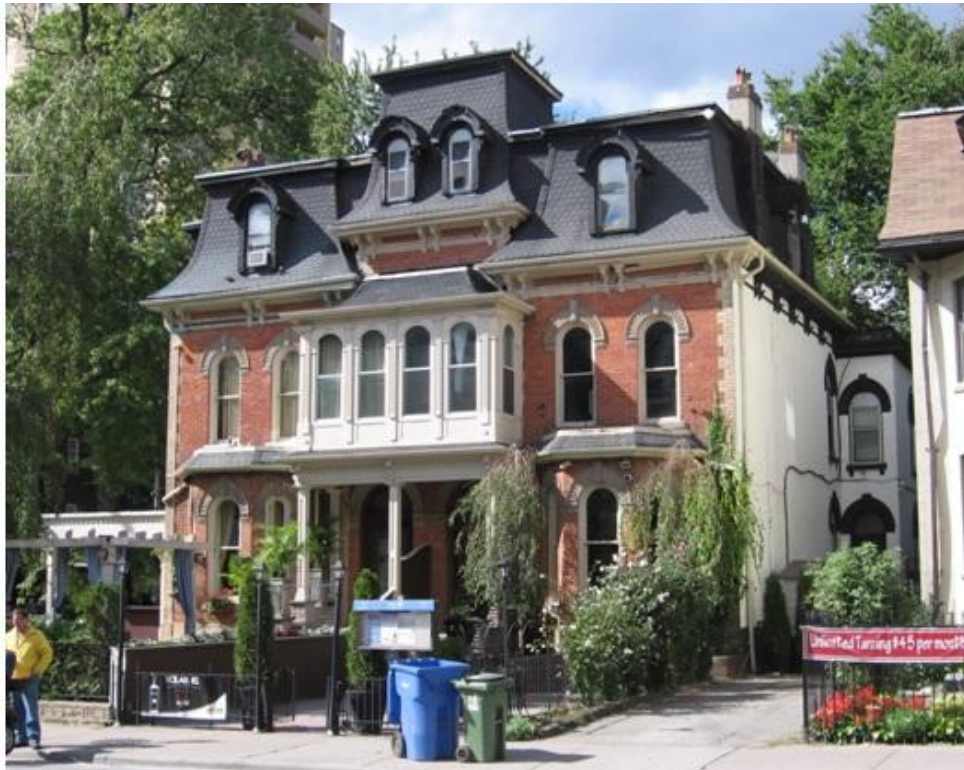
16. Photographs, Church Street Neighbourhood, 2011 : south of the subject properties, the designated heritage properties at 580 (582) Church Street adjoining the northwest corner of Dundonald Street contain other examples of surviving house form buildings on Church Street that share the vintage and Second Empire styling of the subject buildings (Heritage Preservation Services).
