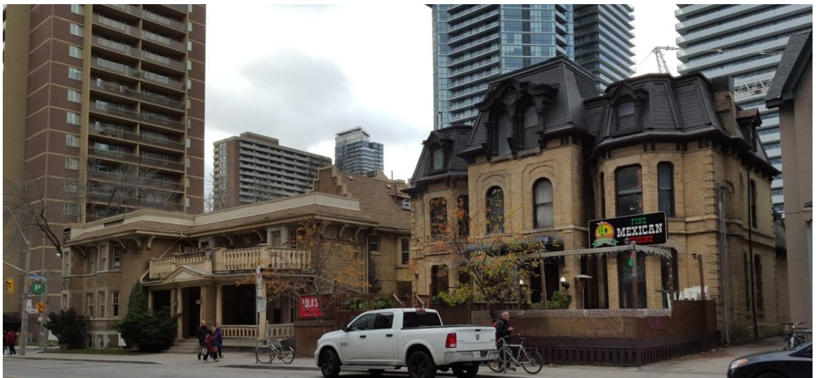
13. Current Photographs, 634 and 636 Church Street, 2016 : contextual views of the properties, looking north on Church Street (above) and south toward Charles Street East (below), and showing the side elevations (north and south) of the semi-detached houses that are viewed from Church Street (Heritage Preservation Services).
