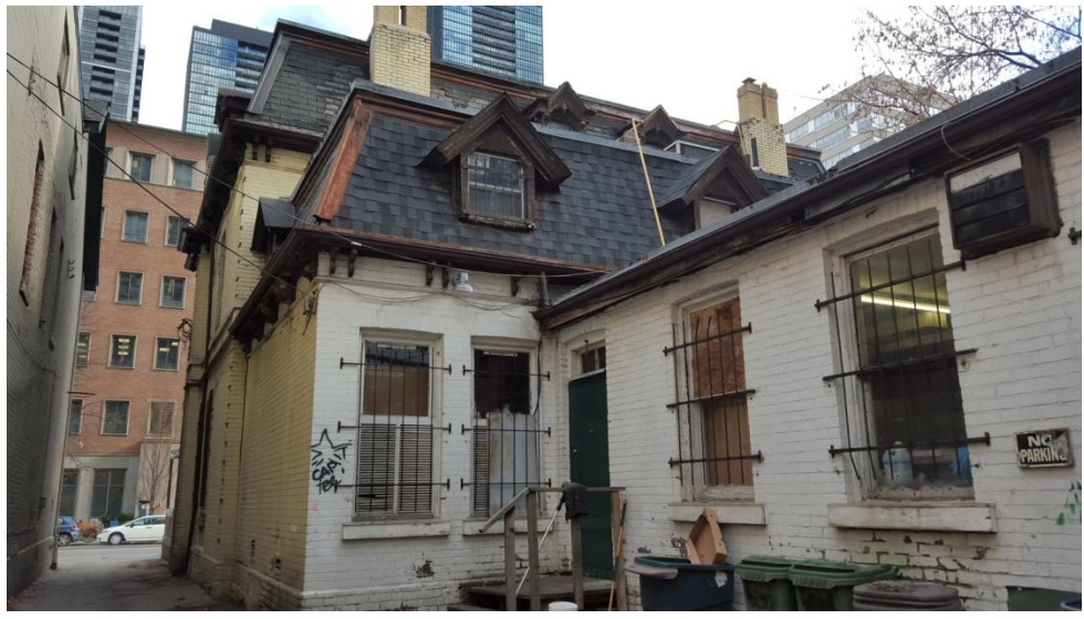
14. Current Photographs, 634 and 636 Church Street, 2016 : detailed view of the north (side) elevation of 634 Church (above) and the rear (west) walls (below) (Heritage Preservation Services).
