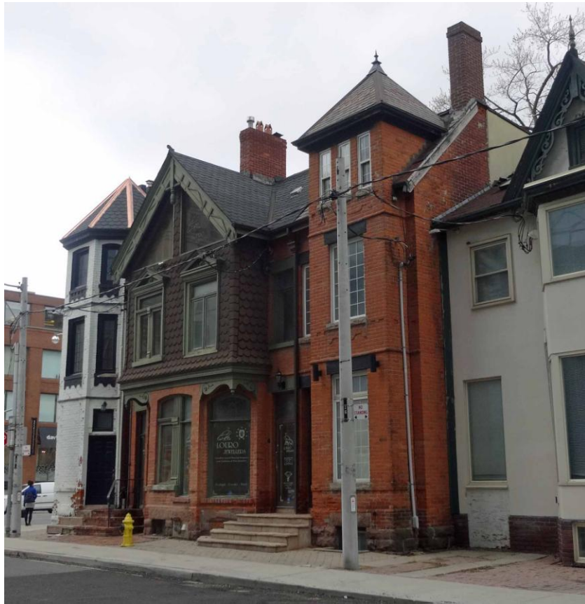
18. Current Photographs, 54A, 56 and 58 Scollard Street and 1315 Bay Street, April 2016 : showing the principal (south) elevations of the row houses (above) and the east (side) elevation of the unit at 54A Scollard (below) (Heritage Preservation Services).
