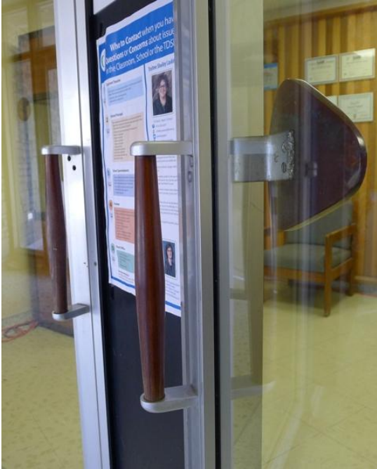
35. Main Entry - Vestibule door pulls (left) : showing the combination of cast aluminum and wood handles (HPS, 2016)
