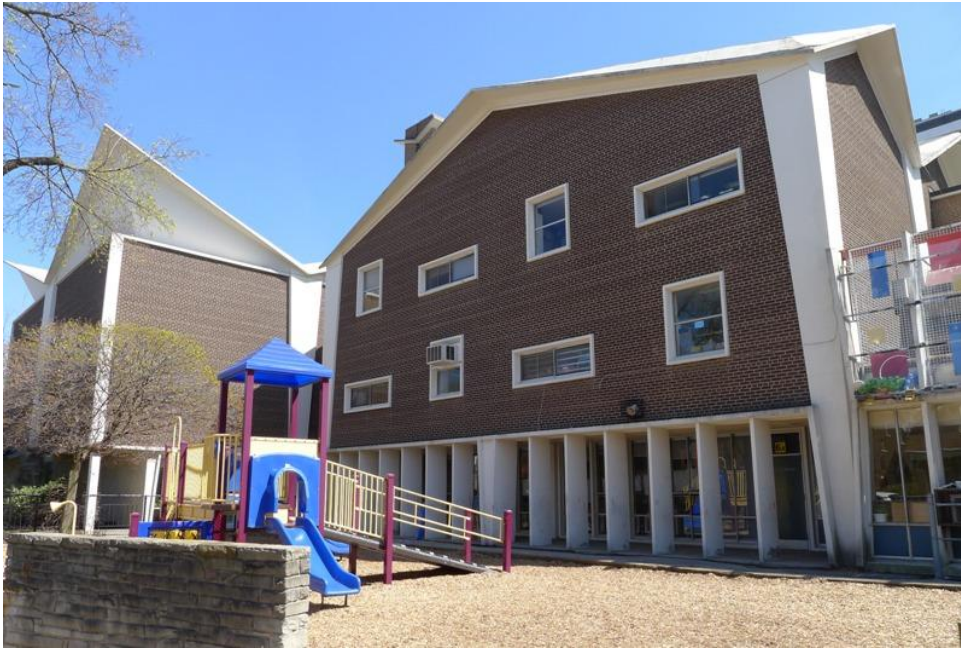
20. Junior School Wing, North Elevation : showing entry pavilion at the left and the house-like form of the pavilion, with first floor 'colonnade' of pre-cast concrete fins and full-length windows extending to the ground providing visual continuity with the playground and the playful arrangement of the windows at the second and third floor levels. In the foreground is an original stone playground wall. ( HPS, 2016 )
