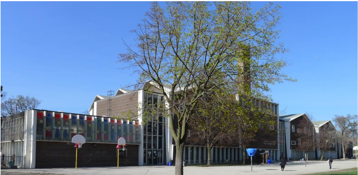
22. South Elevation of the School facing the Playground : showing the day nursery with roof top playground, on the left, and the assembly of pavilions with linking elements enclosing stairs or other services in between. (HPS, 2016)
