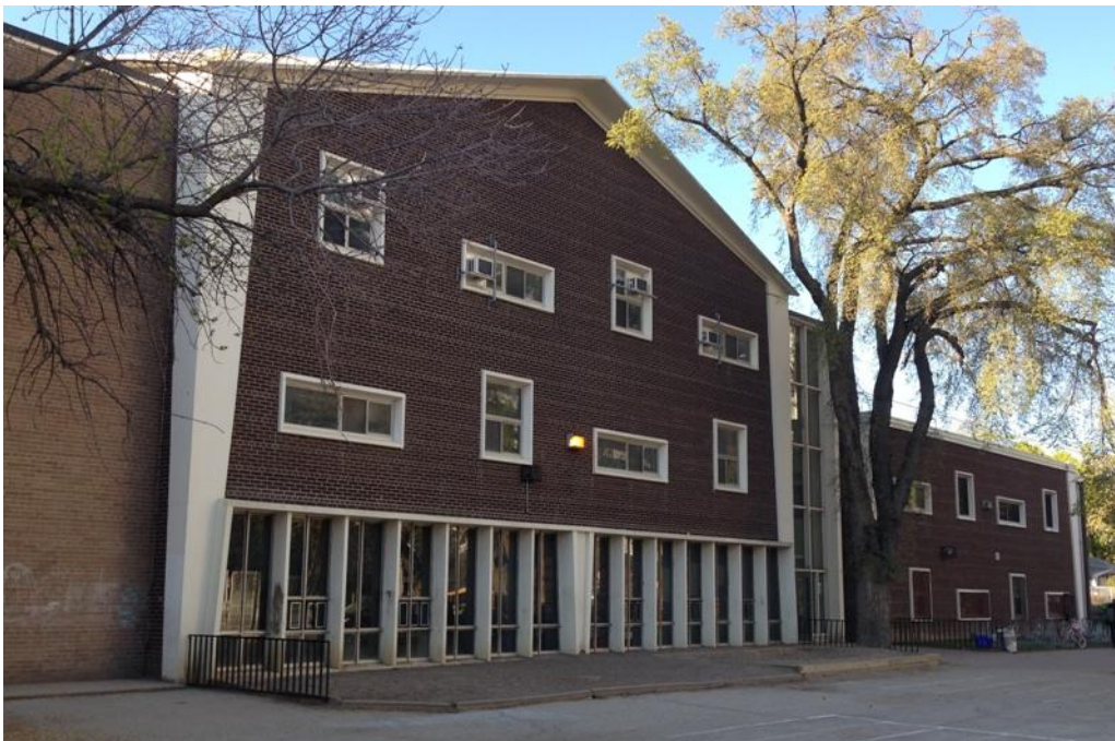
28. South Elevation with 1965-6 Addition (far right) : showing one of the original School for the Deaf pavilions with the linking elements which are either in the lighter, buff brick cladding or fully-glazed staircase elements, and at the far right the 1965-6 addition which lacks the gable-roof form, the parabolic roof and is set on the ground without the 'colonnade' of full-height windows. (HPS, 2016)
