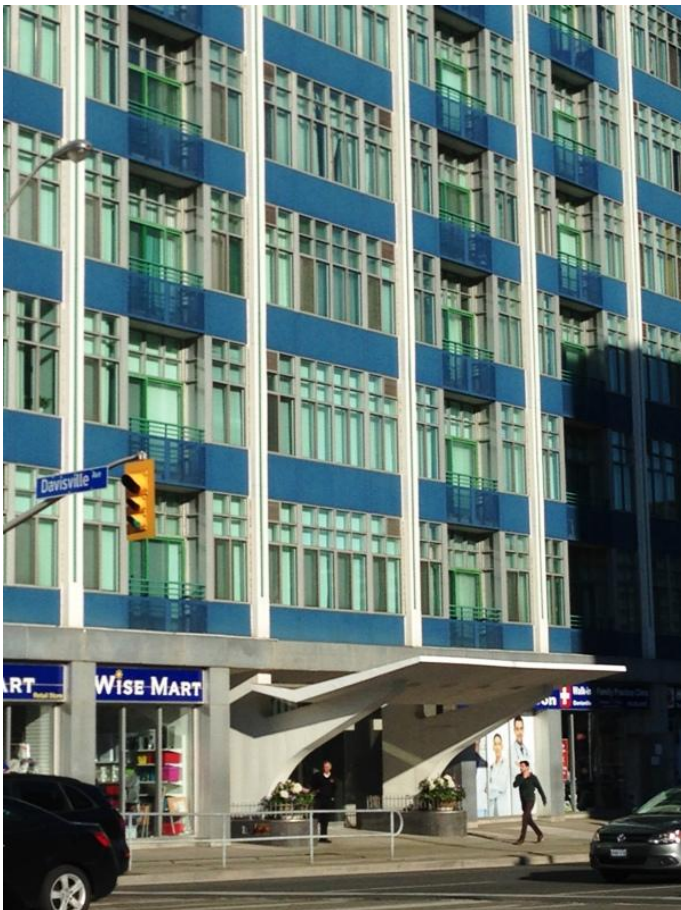
49. High-Rise, c 1960, South-East Corner of Yonge Street and Davisville : showing the Modern Expressionist style prevalent in the Davisville neighbourhood and evident in the dramatic concrete canopy (HPS, 2016)
