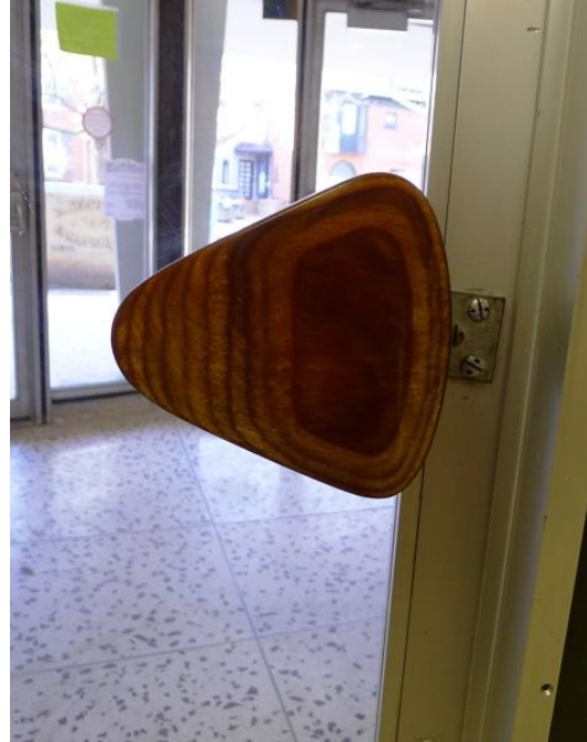
35. Main Entry - Vestibule door pulls (left) : showing the combination of cast aluminum and wood handles (HPS, 2016)
