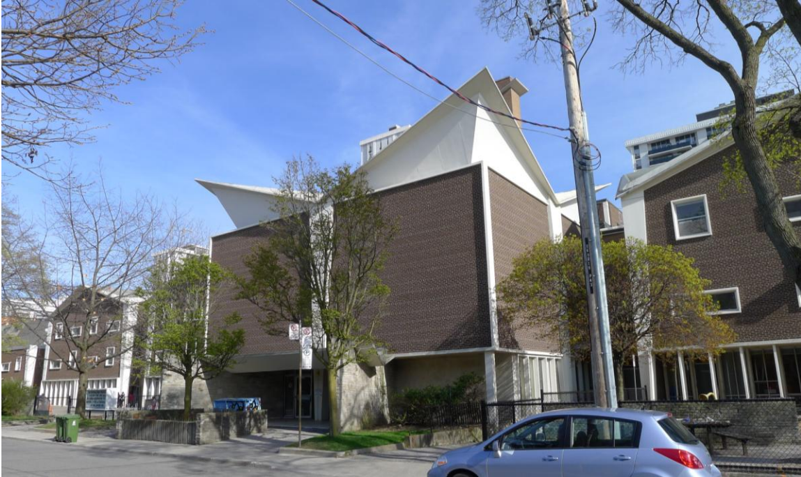
15. North Elevation of the Metropolitan Toronto School for the Deaf and the Davisville Junior School, 1962 facing Millwood Road: showing the central entry pavilion with its dramatic four-corner inverted roof, the Junior School on the right and the School for the Deaf at the left. (HPS, May 2016)
