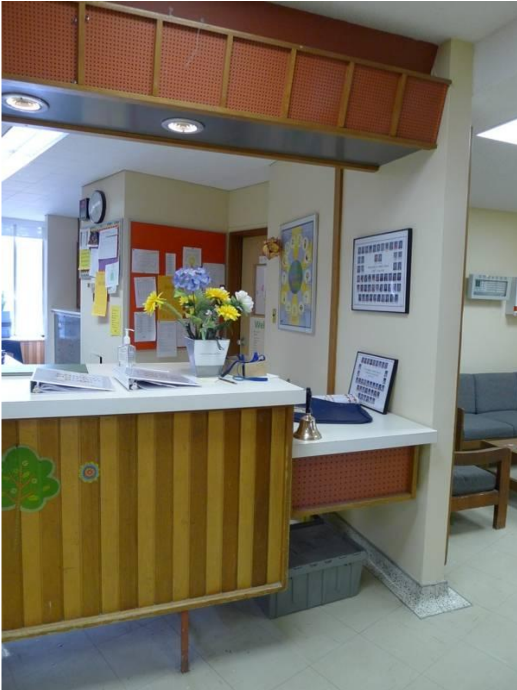
38. Entry Lobby Counter : showing the details with the lower level counter for the children with the red perforated masonite, the two-tone striped desk, the original lighting with the red masonite and soffit in blue (HPS, 2016)
