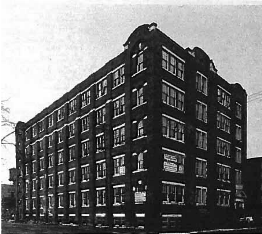
11. Archival Photograph, “Construction” Magazine, May 1909 : showing the Southam Press Building on the southeast corner of Duncan Street (right) and Adelaide Street West (left) following its construction, with the semi-elliptical pediments in place on the rooflines.
