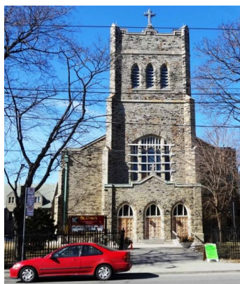
Fourplex at 588-594 Markham Street (above left); Wrigley Brothers' Grocery Store at 585 Bloor Street West (above right); St. Peter's Roman Catholic Church at 840 Bathurst Street (below) (Heritage Preservation Services, May 2015)
