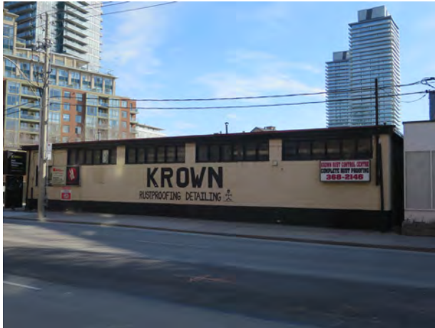
FIG 36 A POST-WAR LIGHT INDUSTRIAL BUILDING FACING ONTO PARLIAMENT STREET (THA 2016).
