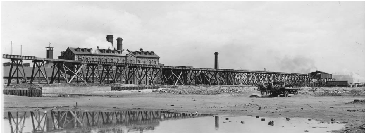
FIG. 19 THE WOOD TRESTLE THAT PRECEDED THE CONSTRUCTION OF THE USRC (CITY OF TORONTO ARCHIVES: FOND 372, SERIES 79, ITEM 209).
