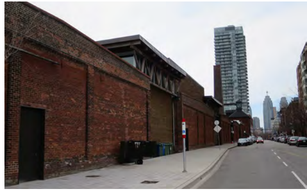
FIG 40 THE INTERNAL NATURE OF THE FORMER INDUSTRIAL SITE IS APPARENT IN THE BLANK FACADES LINING THE SOUTH SIDE OF MILL STREET (THA 2016).
