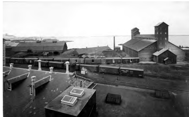
FIG. 18 A 1918 VIEW OVER THE SOUTH END OF THE GOODERHAM & WORTS FACILITIES, SHOWING ELEMENTS THAT WERE DEMOLISHED WITH CONSTRUCTION OF THE USRC (CITY OF TORONTO ARCHIVES: FONDS 1583, ITEM 64).
