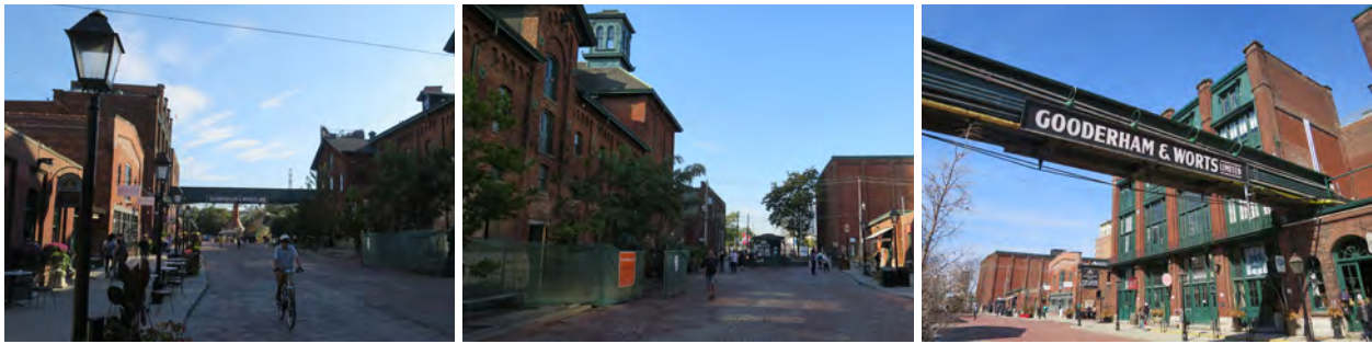
FIG 33 - 35 THE CONCENTRATION OF INTERIOR ADAPTIVE RE-USE BUILDINGS ALONG TRINITY STREET CREATES AN HISTORIC INDUSTRIAL STREETScape OF HIGH LEGIBILITY (THA 2016).
