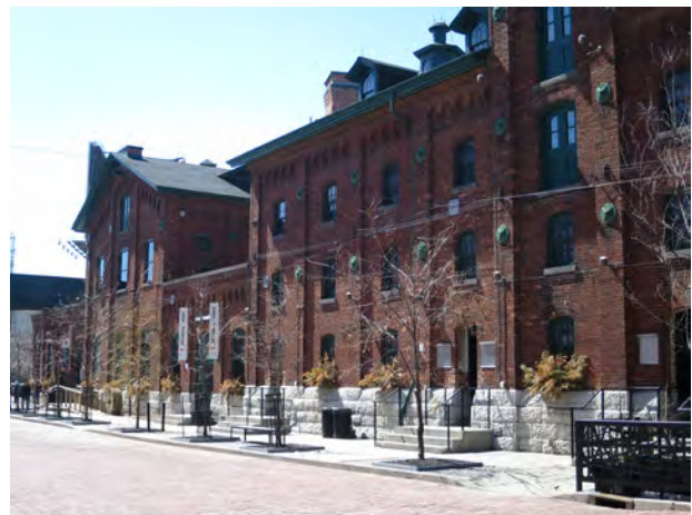
FIG. 21 THE COOPERAGE AND MALTINGS GROUP PRESENTS A CONSISTENT ARCHITECTURAL VOCABULARY TO TRINITY STREET, MASKING THE DISTINCT FUNCTIONAL SPACES WITHIN (THA 2016).
