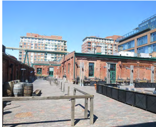
FIG. 24 THE REGULAR GRID ARRANGEMENT OF SINGULAR FUNCTION BUILDINGS IS APPARENT LOOKING NORTH UP PURE SPIRITS MEWS (THA 2016).
