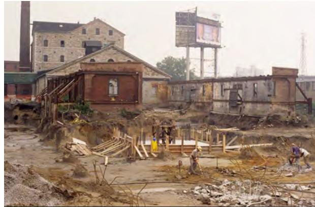
FIG. 14 RENOVATIONS UNDERWAY AT THE MACHINE SHOP (BLDGS. NO. 8, 9) c.1990 (CITY OF TORONTO ARCHIVES: SERIES 1465, FILE 3, ITEM 14).
