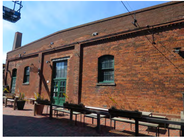
FIG. 23 TANK HOUSE 4 EXHIBITS THE SCALE, MASSING AND SIMPLE ARCHITECTURAL LANGUAGE TYPICAL OF MOST SINGULAR FUNCTION BUILDINGS (THA 2016).
