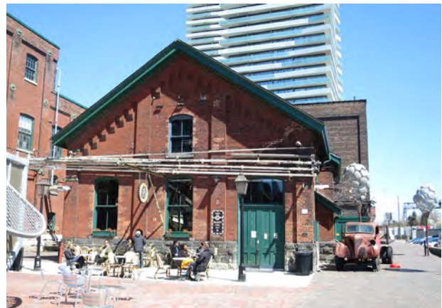
FIGS. 26 - 29 THE DIVERSE FORMS AND SIZES TYPICAL OF OPERATIONS SUPPORT BUILDINGS, AS SEEN (FROM TOP TO BOTTOM) IN THE WORKSHOPS, LUNCH ROOM, CASE GOODS WAREHOUSE, AND PUMP HOUSE (THA 2016).
