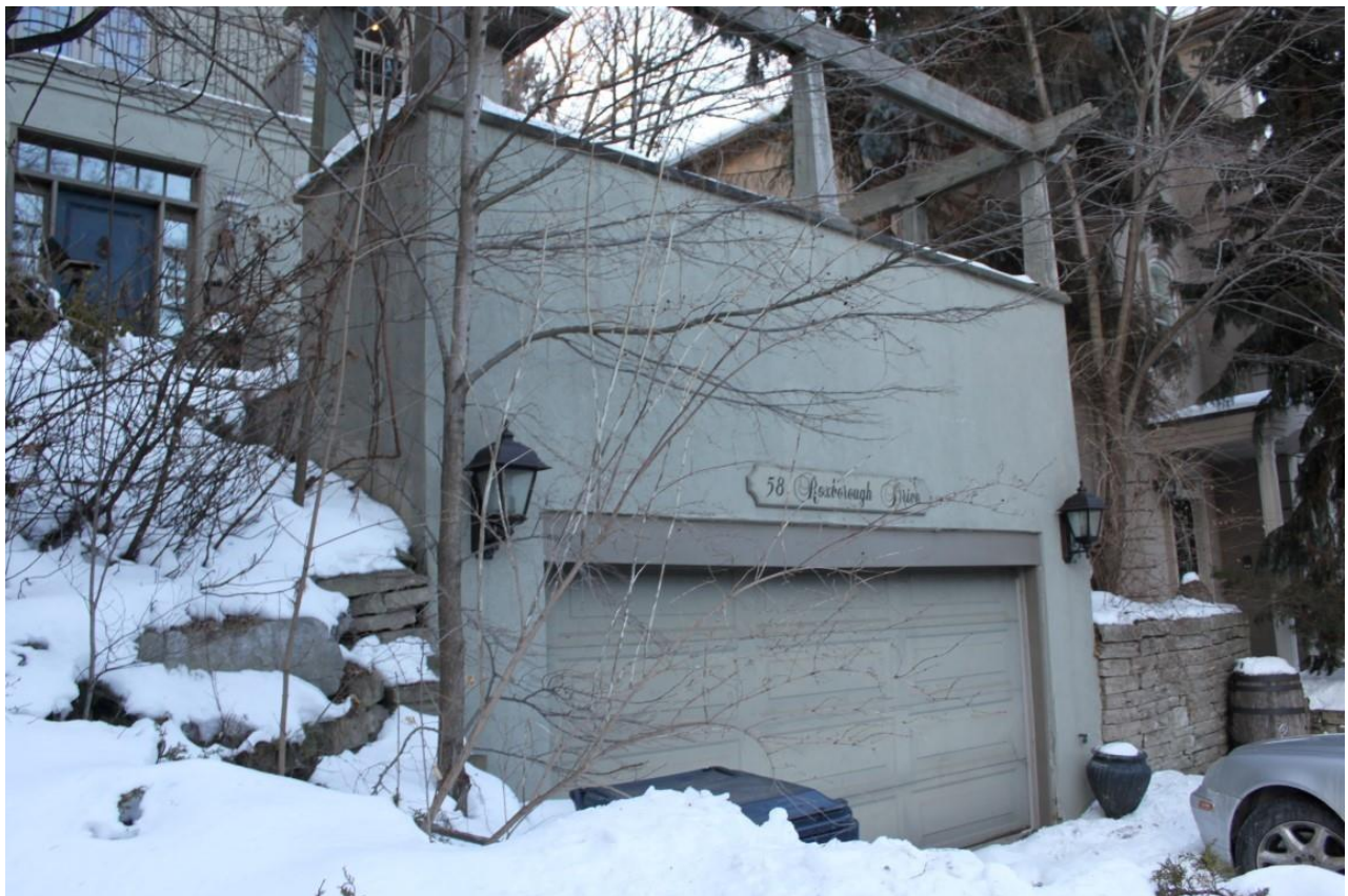
The existing garage is below grade and classified as legal non-conforming.
