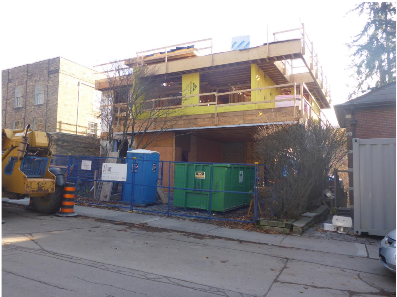
Current construction on Roxborough Drive after demolition of unrated home.
