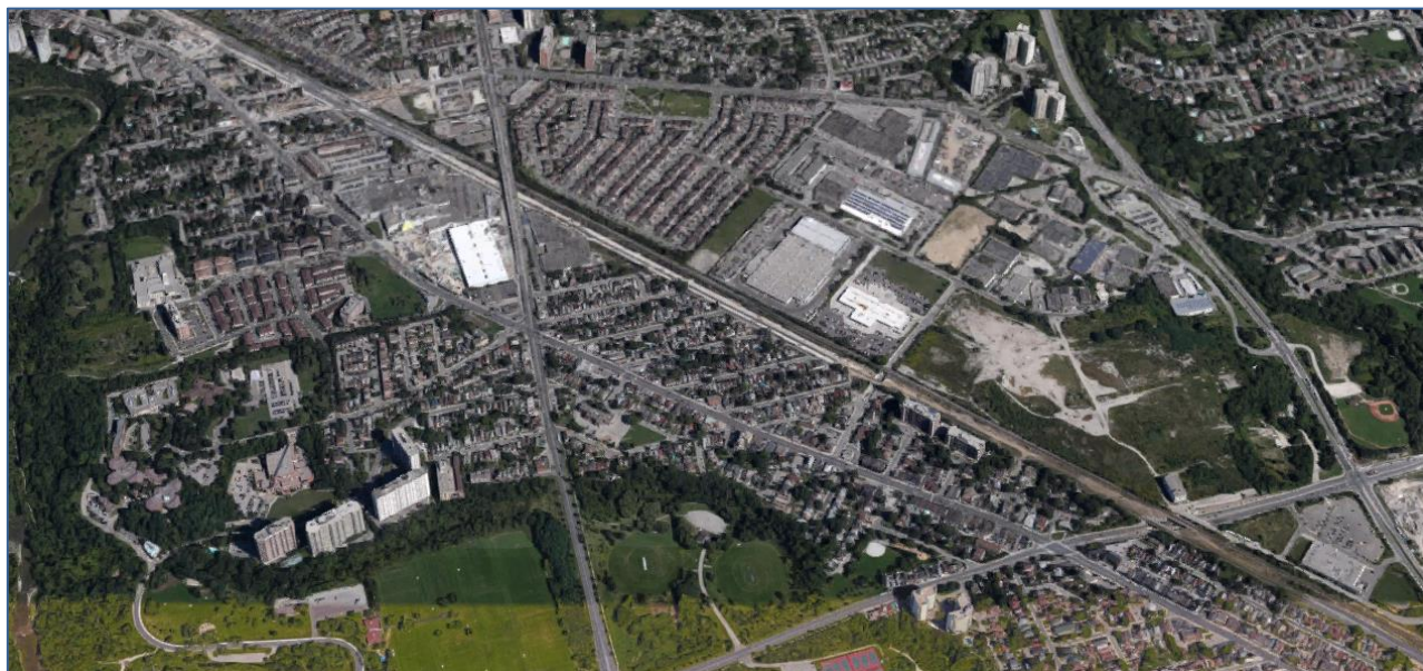
Figure 2. Mount Dennis existing buildings. (Google Maps)
