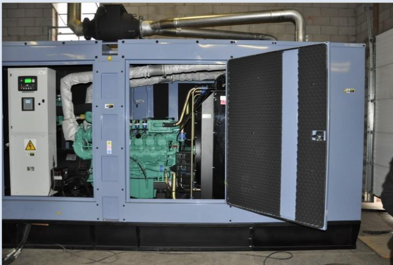
Packaged, 400 kW natural gas-fired generator.
