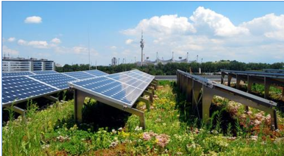
Figure 11. Solar PV installation on a green rooftop installation in Munich, Germany 9 .
