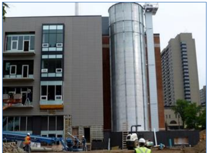
Figure 12. Wood pellet storage silo integrated with residential buildings in La Cite Verte, Quebec City. 10
