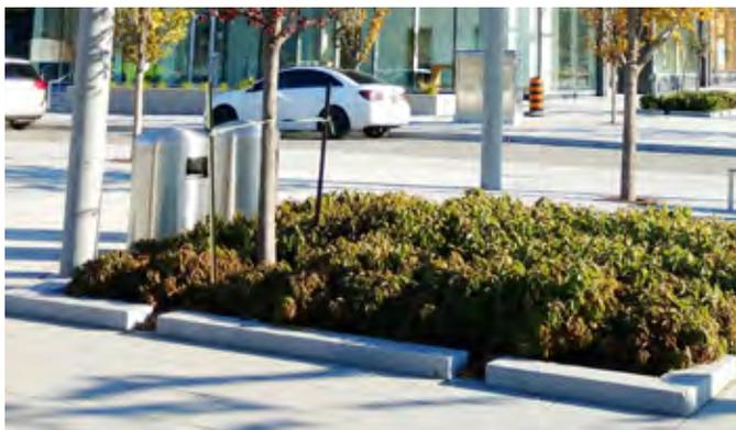
Figure 1: Front Street, West Don Lands - stormwater directed into landscape bed curb openings.
