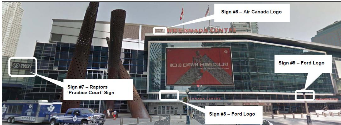
Figure 11 – West facing elevation of Air Canada Centre
