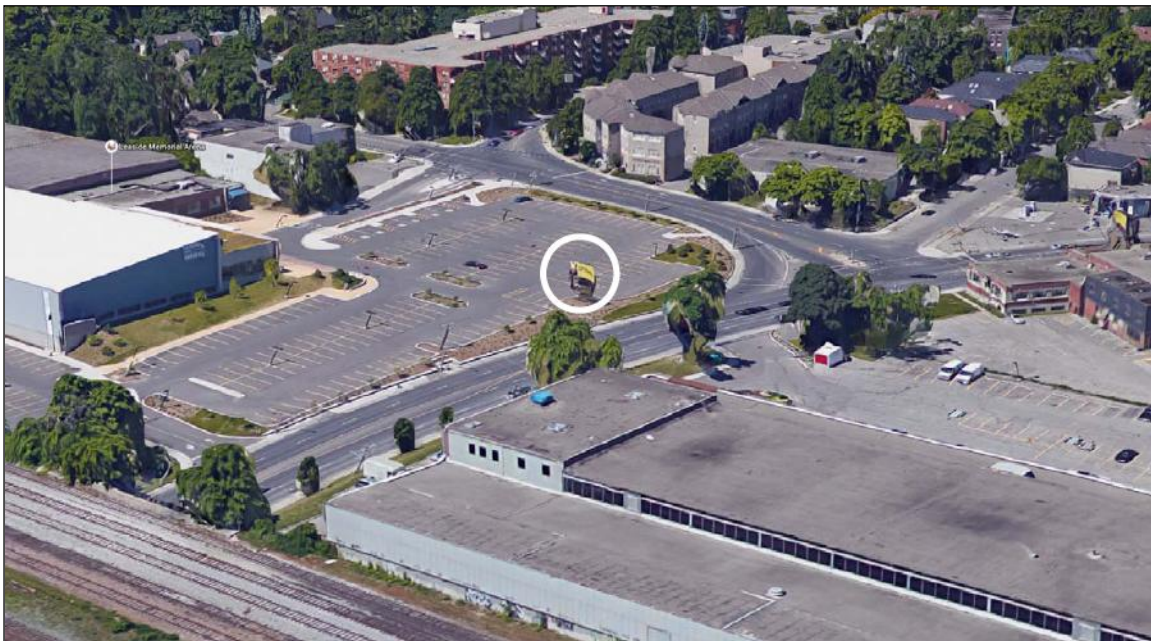
Figure 2 – View of third-party sign to be replaced at Leaside Memorial Gardens and surrounding area (looking north-west)
