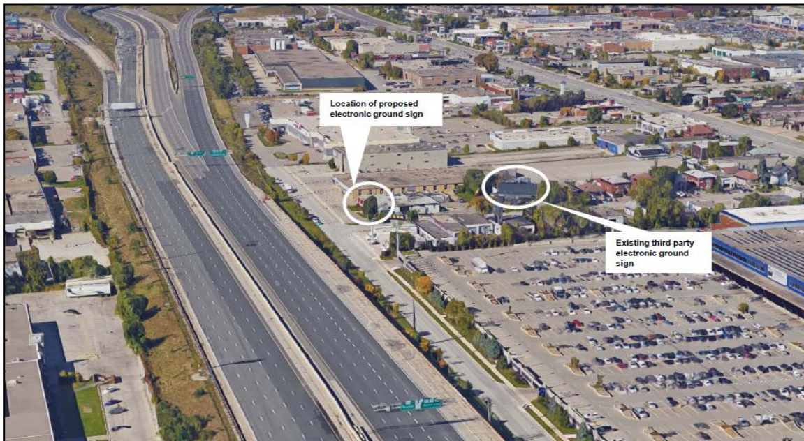
Figure 4 – 64 Fordhouse and surrounding area (looking west along the F.G. Gardiner Expressway)
