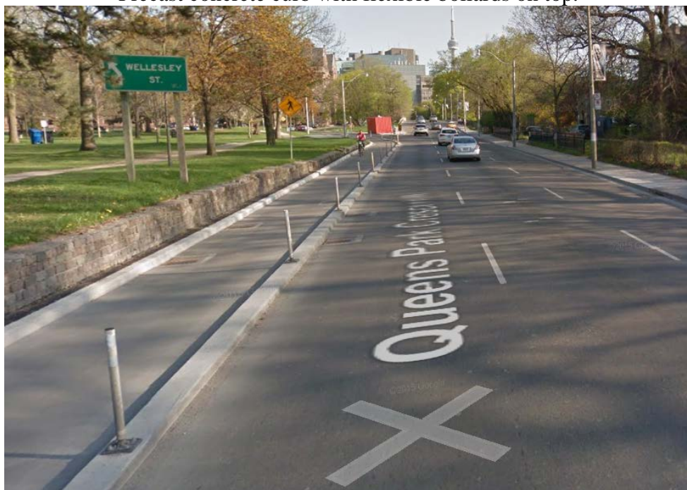
Precast concrete curb with flexible bollards on top.
