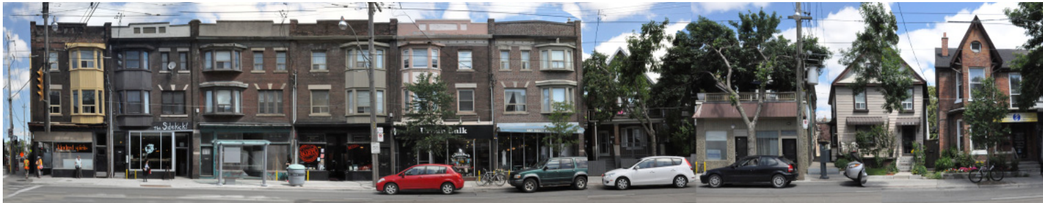
Queen Street East (Greenwood Avenue to Vancouver Avenue)
