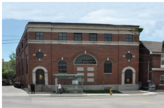
1353 Queen Street East
