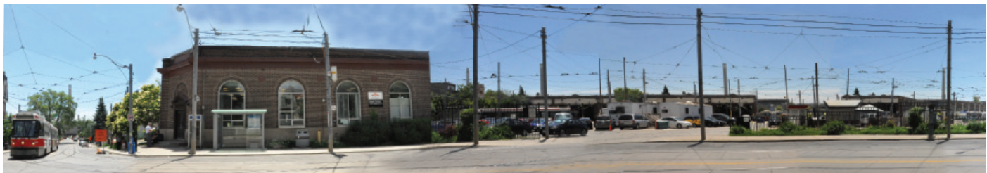
TTC Russell Division (Connaught) Streetcar Barns carhouse building at 1433 Queen Street East
