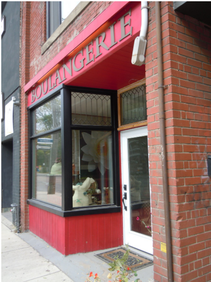
The at-grade condition of buildings, including glazing, signage and materials is critical to the character of the public realm.
