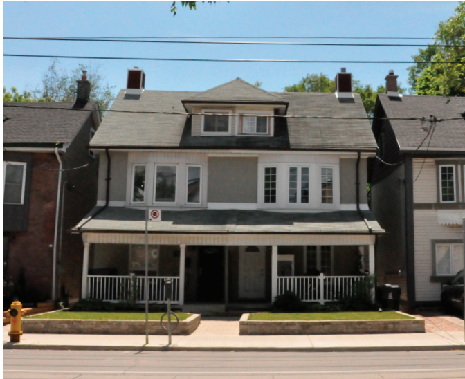
The photo above illustrates the residential front yard setback condition that exists in several locations within the study area; some of these setbacks are landscaped (shown at centre), while others are paved or used as parking pads.
