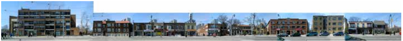
West of Broadview Avenue, from Danforth Avenue to Pretoria Avenue
