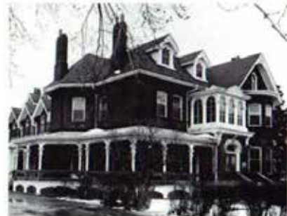
Chester Park, demolished ( East York Historical Society )
