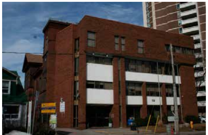
Chester Public School at 958 Broadview Avenue was converted to the Estonian House in the 1960s and has remained a cultural hub for the Estonian Canadian community since. The front addition was added in the 1970s. The property was included on the Heritage Register in 2006.
