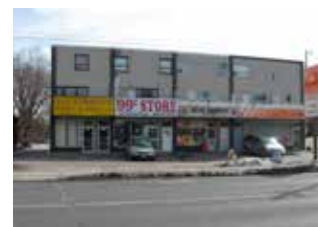
Bater's General Store site at 1129 Broadview Avenue, 2015
