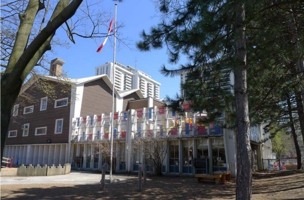
25. Day Nursery Wing : showing the roof top playground at the second level with colourful panels on the enclosure. The Junior School is at the left of the photograph. (HPS, 2016)
