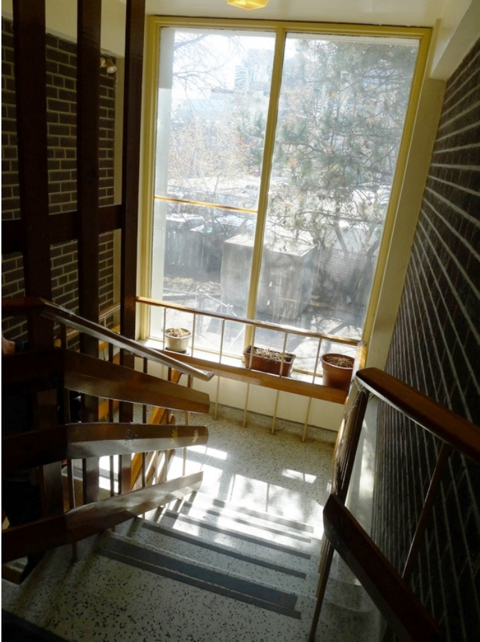
46. Day Nursery Staircase : showing the stairs which are built into the walls and the multiple handrails for additional safety. (HPS, 2016)
