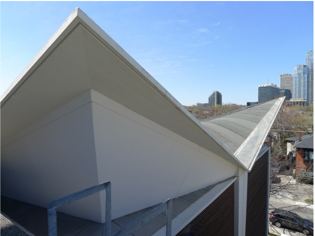
18. Central Entry Pavilion Roof – side view : showing the side elevation and a portion of the edge of the central roof. (HPS, 2016)
