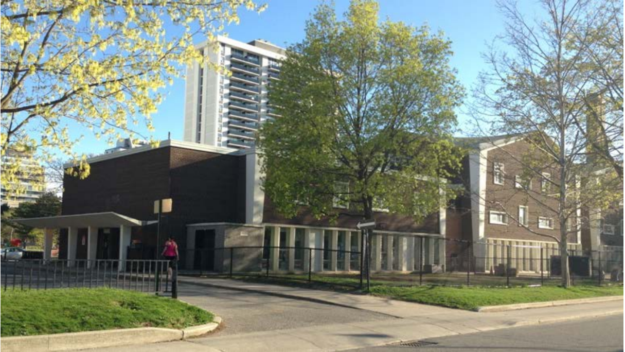
27. Two-Storey Addition, Hicks, Marsh and McLean architects, 1965-6 : showing the east and north elevations with the ground floor full-height windows with 'colonnade' feature and window pattern of the original school building and the entry canopy for vehicle pick-ups and drop-off. The pavilion for the School for the Deaf is at the right (HPS, 2016)
