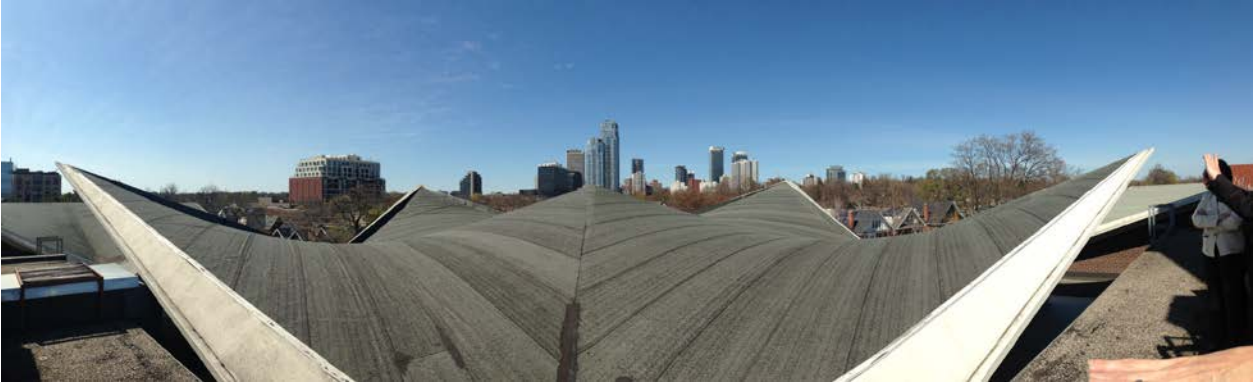
17. Central Entry Pavilion Roof : showing the sculptural form and materials of the roof top (HPS, 2016)
