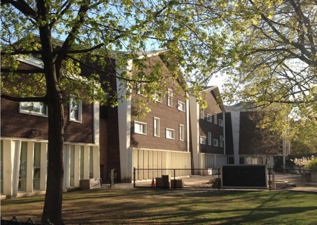
21. School for the Deaf, North Elevation : showing the 1965-6 addition on the left with the two pavilions for the School for the Deaf in the centre and the projecting entry pavilion at the right. As at the junior school the ground floor colonnades of thin concrete fins and full-length windows provide continuity with the exterior and a more domestic scale is maintained at the upper floors. (HPS, 2016)
