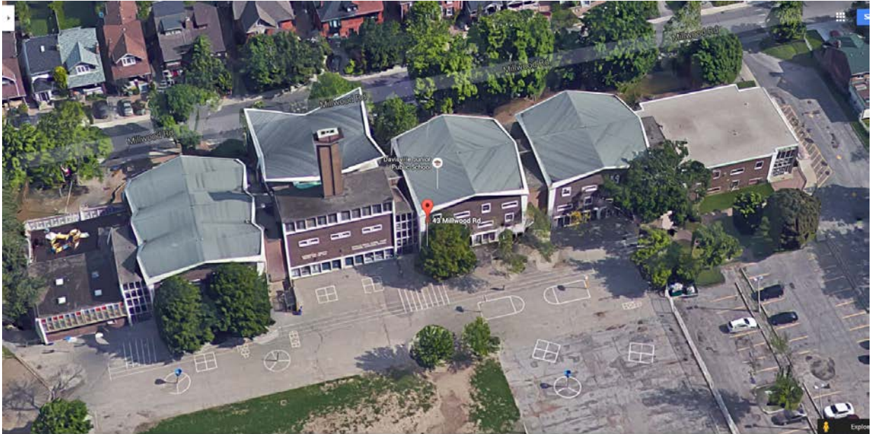
16. Aerial photograph of the 1962 school from the south: showing the south elevations facing the playground with the day care centre and junior school on the left, the entry pavilion behind the chimney in the centre and the school for the deaf on the right, the 1965-6 addition at the extreme right with the flat roof. (Google Maps, April 2016)
