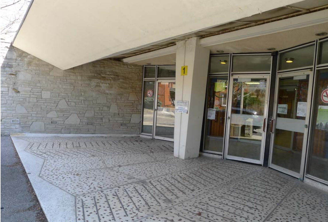
32. The Main School Entrance : showing the inverted concrete canopy, the pier separating the two entrances for the two schools, the zig-zag pattern of the doors with the corresponding zig-zag patterns in the terrazzo and one of two field stone walls framing the entrance with the various sized stones. (HPS, 2016)
