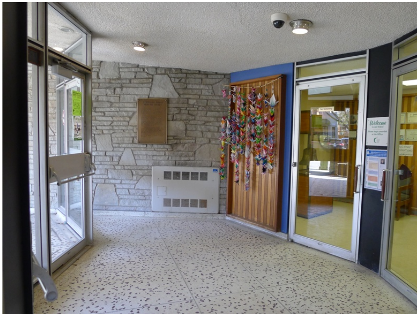
33. Main Entry Vestibule : showing the field-stone wall and terrazzo floor of the exterior continuing into the vestibule where they are combined with the two-toned wood panels of the lobby space (HPS, 2016)
