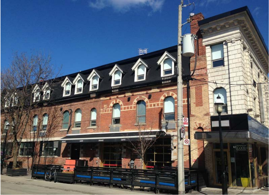
12. 1150 Queen Street West : showing the partially restored west elevation revealing the original buff and red brick patterning of the second to fourth bays from the corner. (HPS, 2016)
