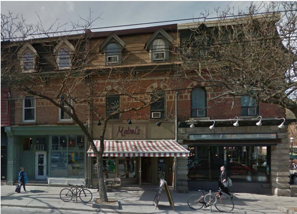
17. 1154-1158 Queen Street West : showing the first three properties of the six on the north-west corner of Queen Street West and Beaconsfield Avenue with matching brick detail on the second floors and the mansard roof with gable-roofed dormers and semi-circular headed. ( google maps, April 2015 )
