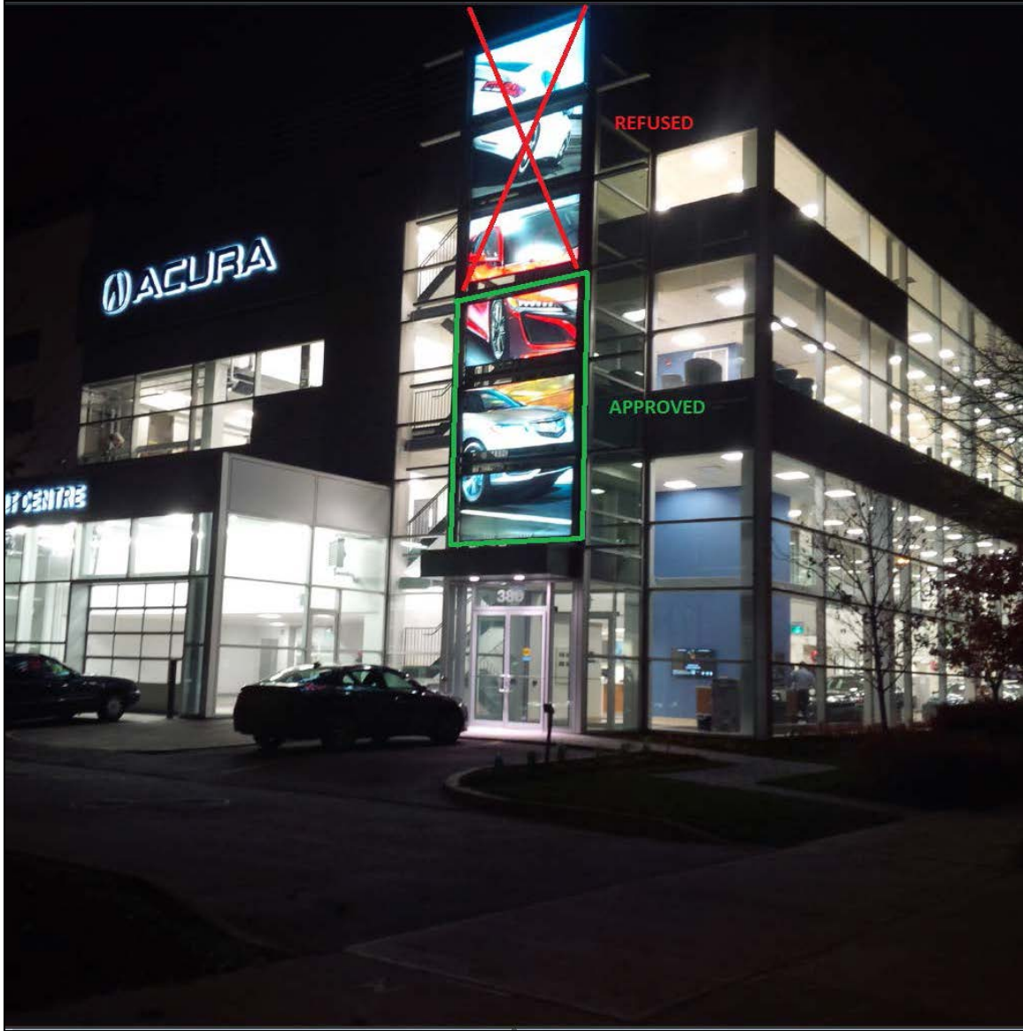
FIGURE A: Signs on Media Tower-type Addition
