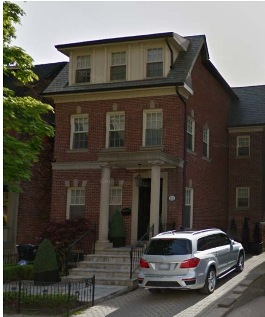
East Elevation of 124 Hazelton Avenue (May 2016)
