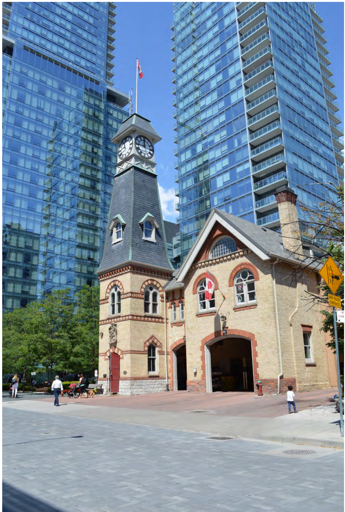
Yorkville Fire Hall (Source: City of Toronto)
