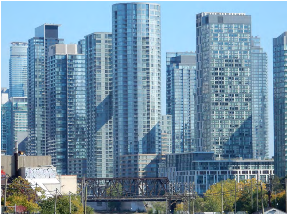
Railway Lands Neighbourhood – an example of a vertical mixed use community (Source: City of Toronto)
