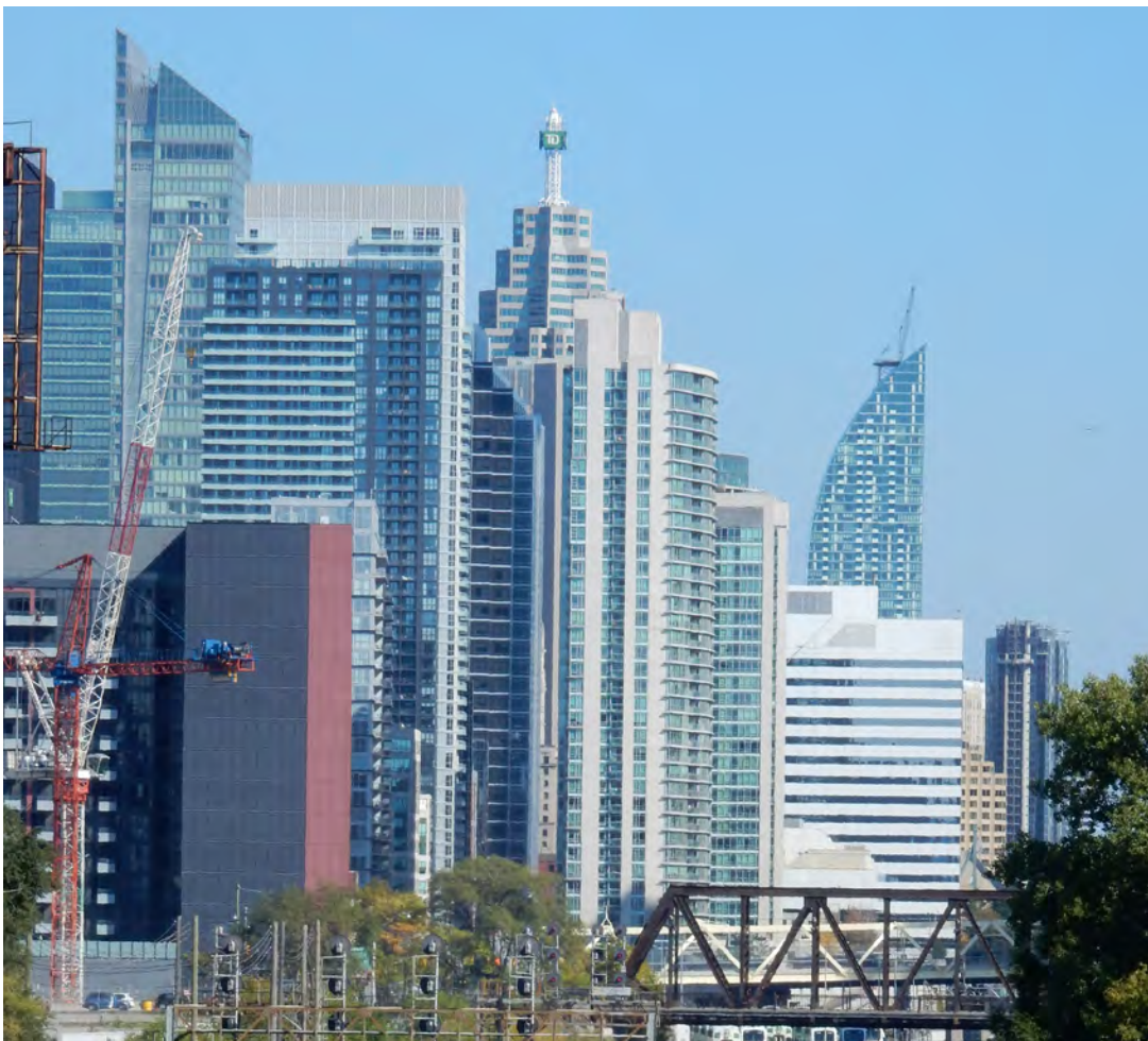
View of the downtown from the west (Source: City of Toronto)
