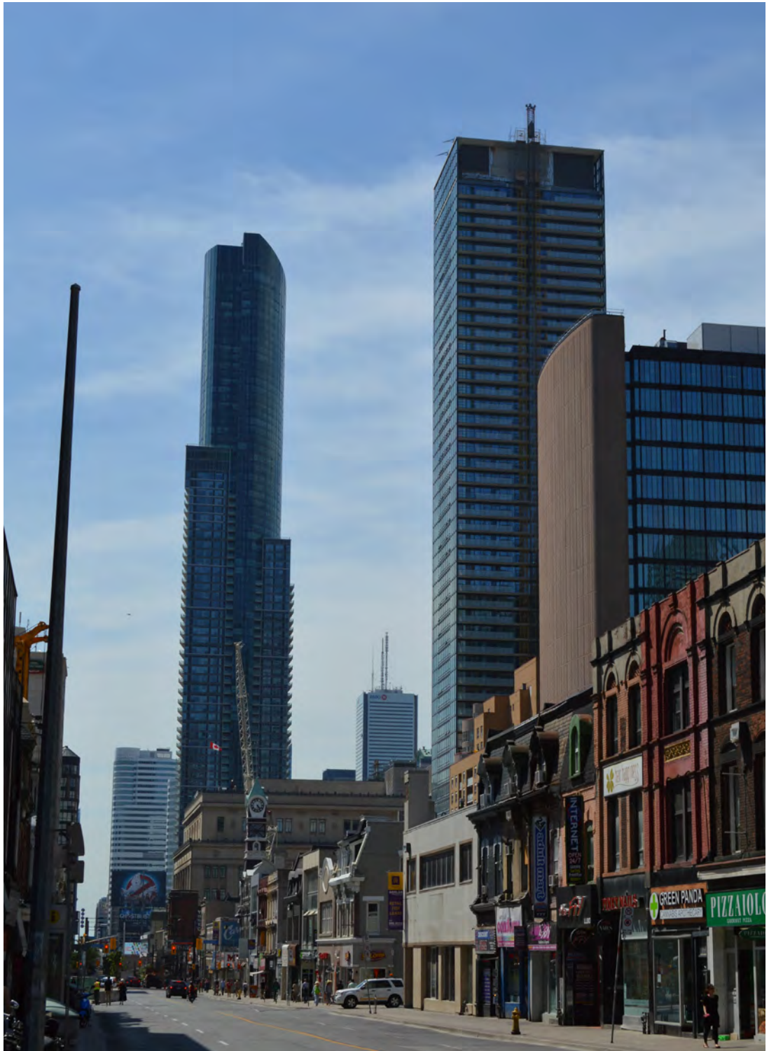
View south along Yonge Street (Source: City of Toronto)
