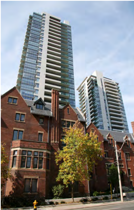
Example of the varied scale of built form Downtown (Source: City of Toronto)
