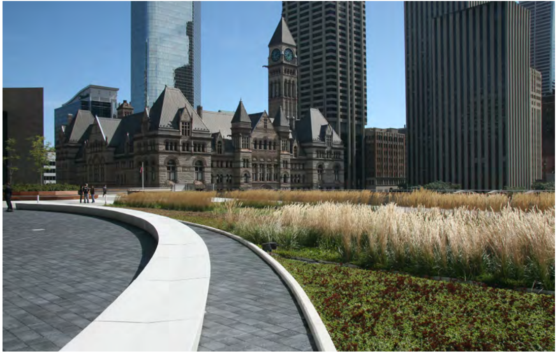
Green Roof at City Hall (Source: City of Toronto)
