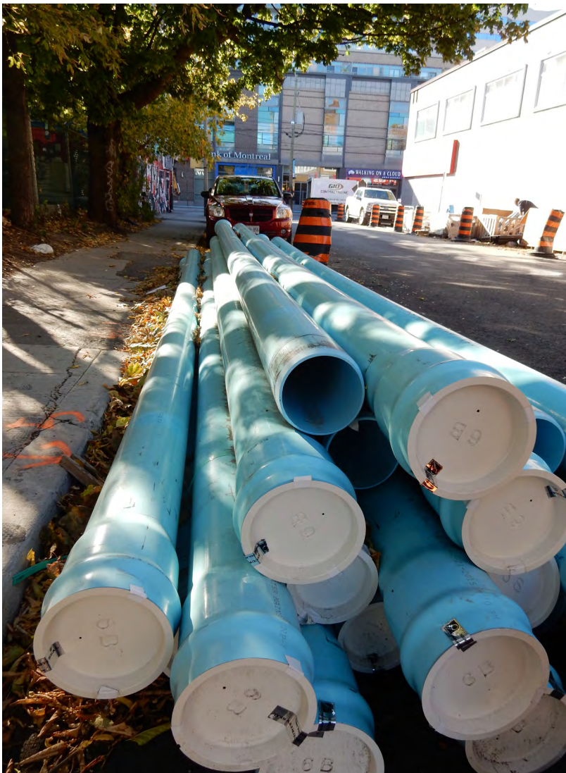
Watermain Replacement (Source: City of Toronto)
