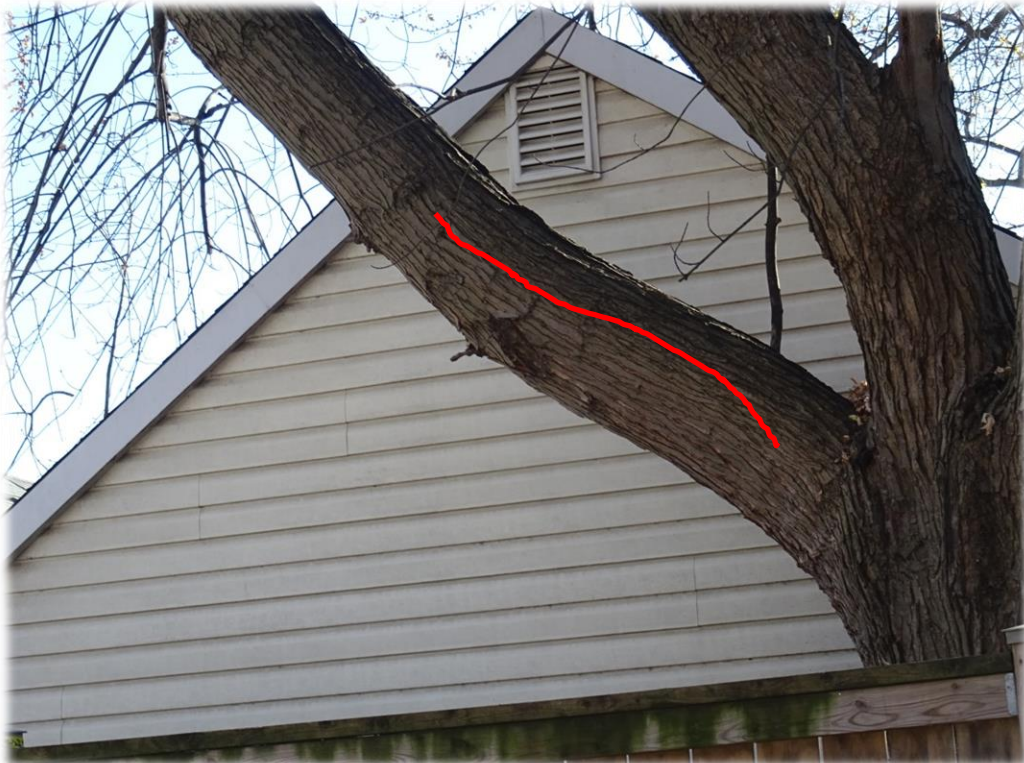
Figure 8: Base of Branch 2 showing crooked shape typical of “hazard beam” failures.
