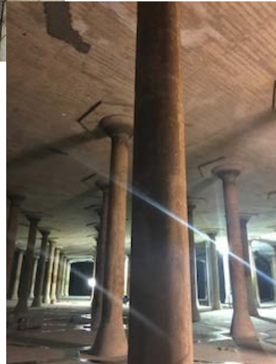
St. Clair Reservoir Rehabilitation
