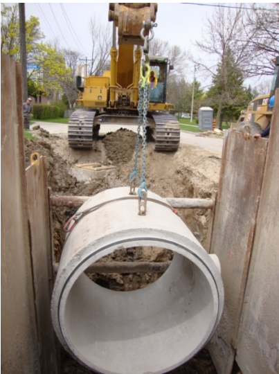
Storm Sewer Upgrades Basement Flooding
