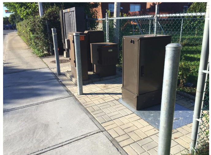
Clustering of equipment – no aesthetic treatment
