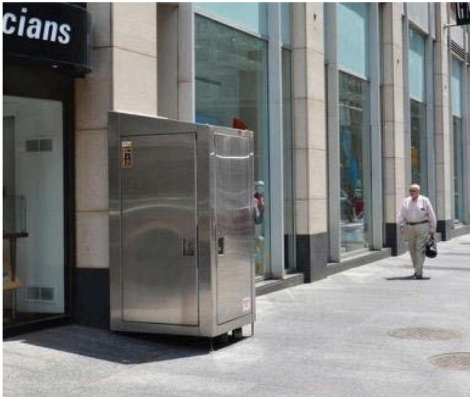
**Photo 6:** Bay & Bloor pipes contained but better placed off the sidewalk in adjacent lane 20 feet away.
