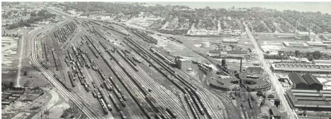
3e. Aerial view east from Mimico Yard to the subject property, 1960s
