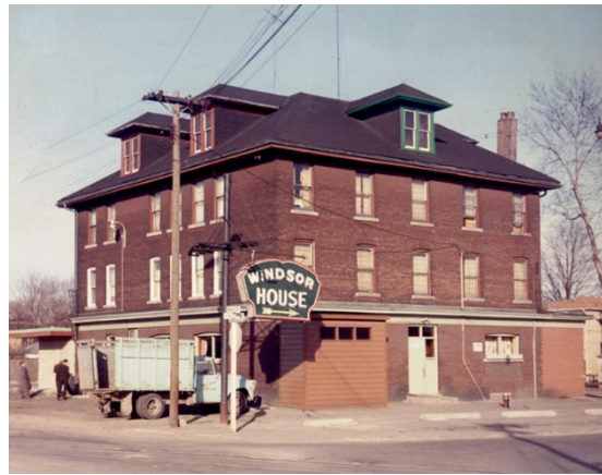
3d. undated photograph with "Windsor House" sign
