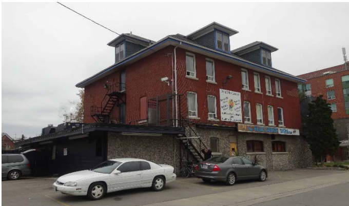
4c. north elevation on Manchester Street, facing the railway tracks (right), with the rear (east) elevation (left)
