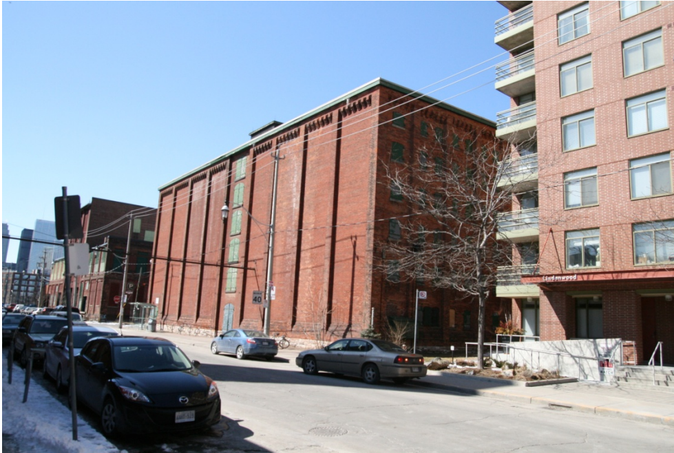
View from South-East Looking North-West
