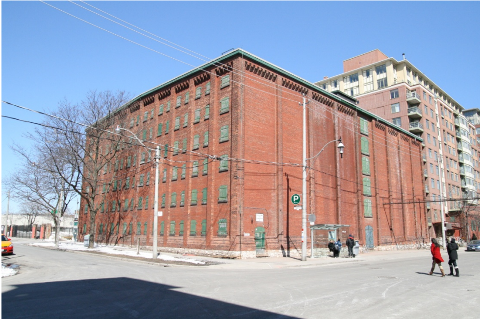
View from South-West Looking North East
