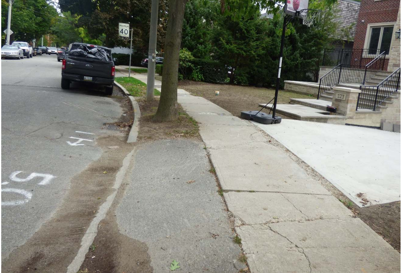
Attachment 2 – TPRR staff photograph of the constructed driveway, existing access way and subject tree.
