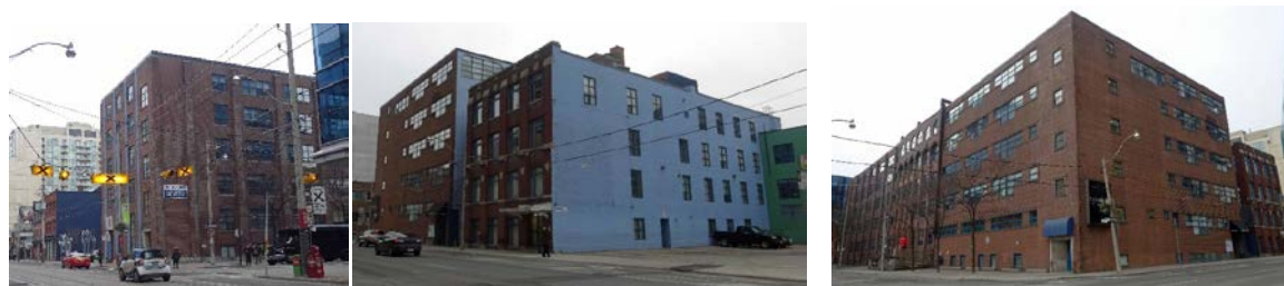
7g, 7h and 7i. Context on King Street East west to Princess Street (left), on Adelaide Street East, east to Ontario Street (centre), and on Ontario Street, south to King Street (right)
