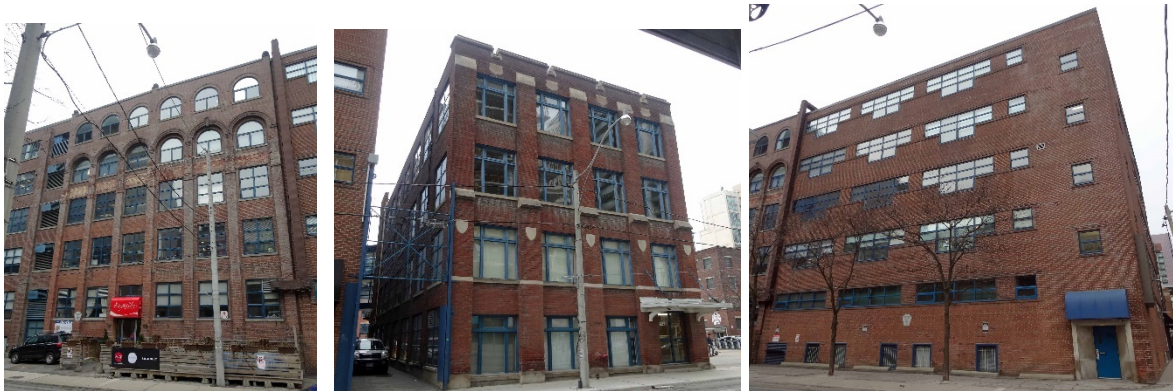
7d, 7e & 7f. 266 King, North Building (left), 427 Adelaide (centre), and 435 Adelaide (right)
