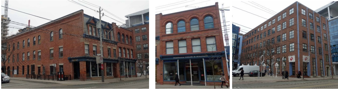
7a, 7b & 7c. 254 King (left), 256 King (centre), and 266 King, South Building (right)
