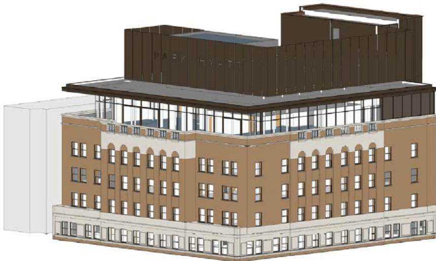
Rendering of the upper section of south tower showing the renovated southeast corner of the new glazed bar and event space with roof top mechanical above.
