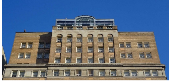
4e. south roofline detailing
