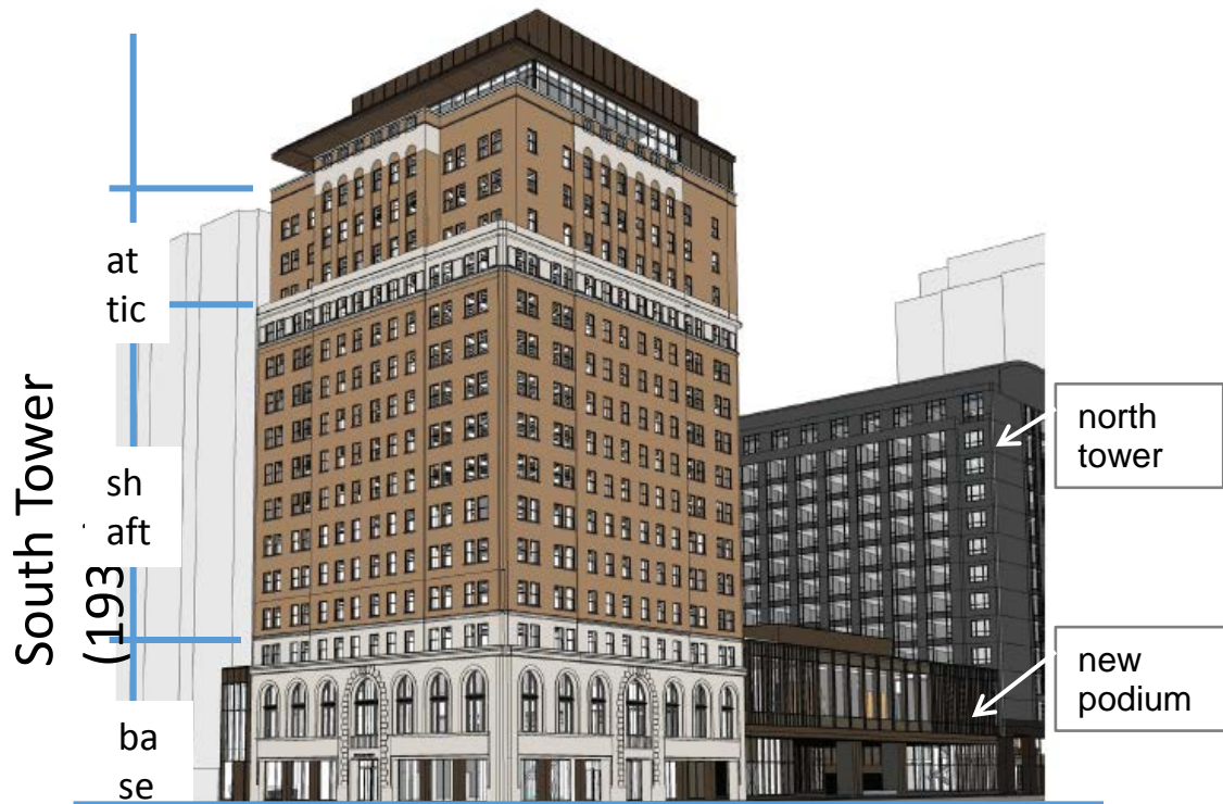
View of the south tower showing the new three-storey retail addition to the west and new podium link to the north tower (right side of image)
