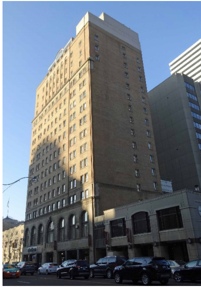
4a. east elevation (left)
