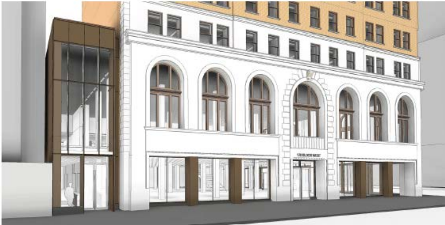
View of the new retail addition connecting with the west side of the south tower as seen from Bloor Street West. The new addition is of contemporary design, set back to reveal the stone quoins and cornice of the existing building.
