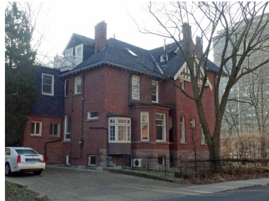
4b. West (right) and north elevations
