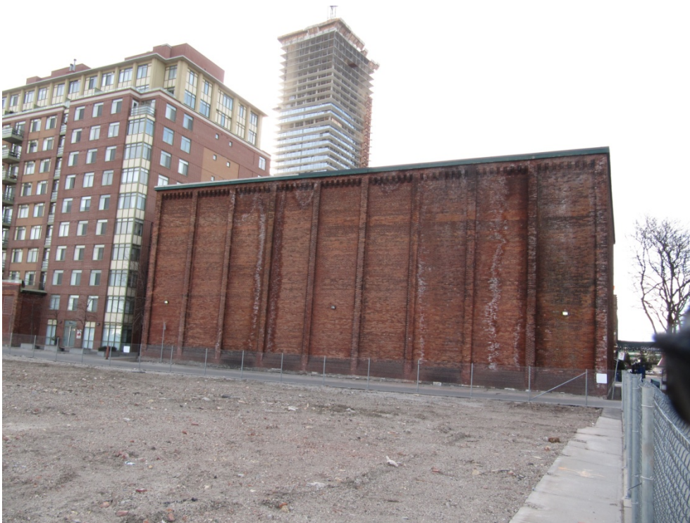
Looking South at North Elevation
