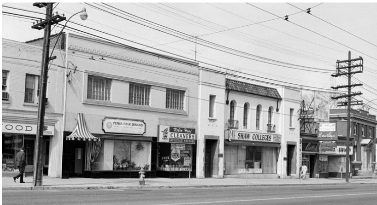
3c. Archival Photograph, 1968: 2430 (left) and 2434 (right) Yonge Street
