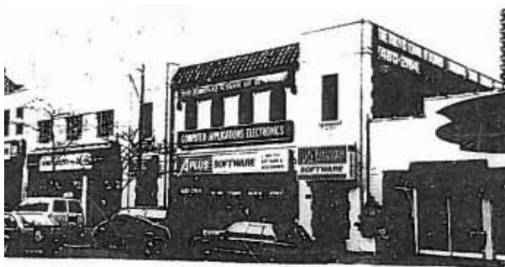
3d. Archival Photograph, 1990: 2430 (left) and 2434 (right) Yonge Street
