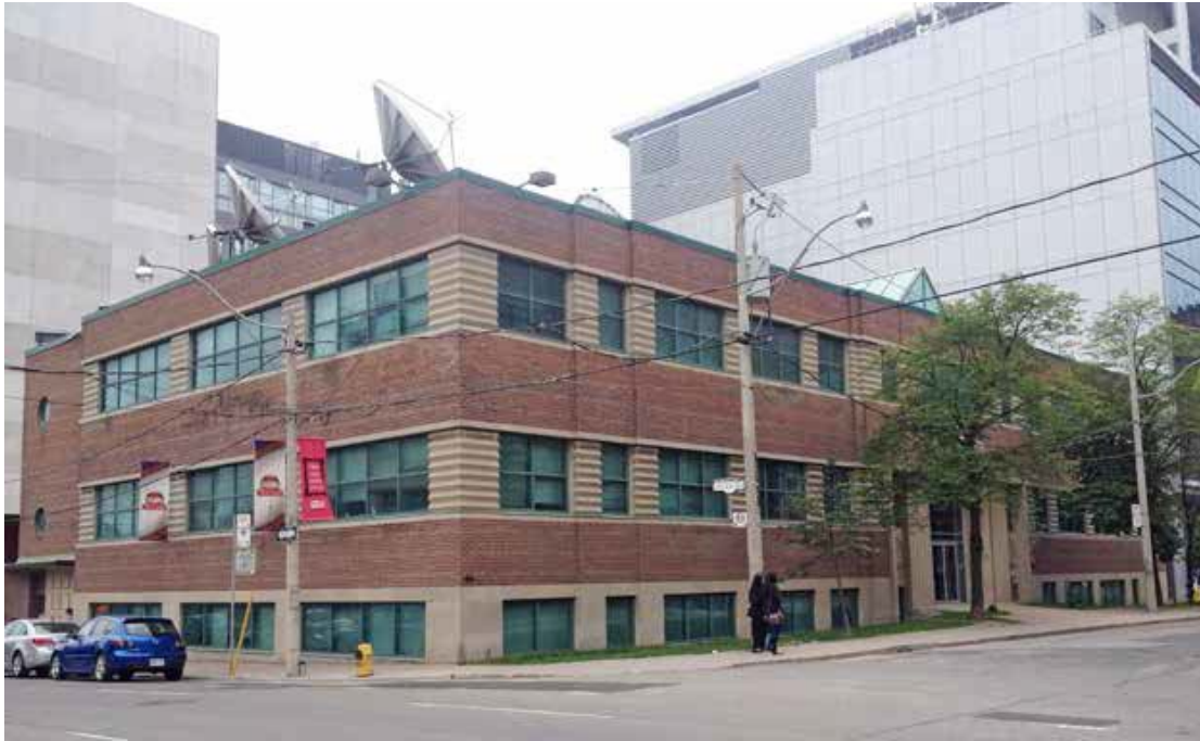
View of 25 Ontario Street showing the Adelaide Street East elevation (left) and the Ontario Street elevation (right) (ERA Architects)
