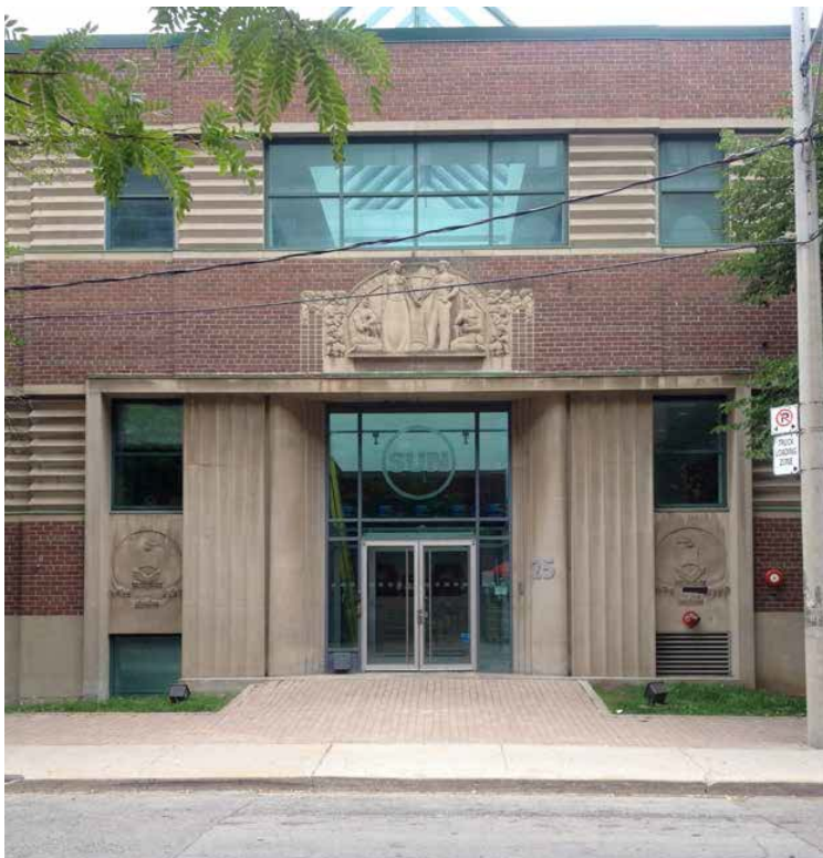
Detail of the principle entrance of Drug Trading Company Administrative Office (ERA Architects)
