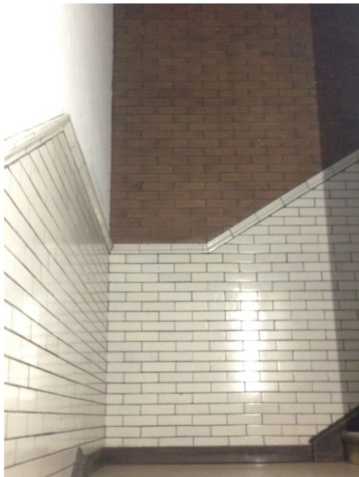
27. Main Stairs showing the glazed tile dado and brick walls above. (HPS, 2017)
