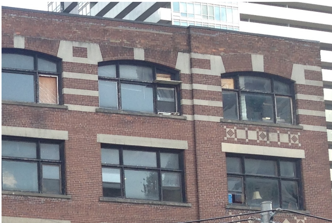
22. Fifth Floor, brick and stone details. (HPS, 2017)
