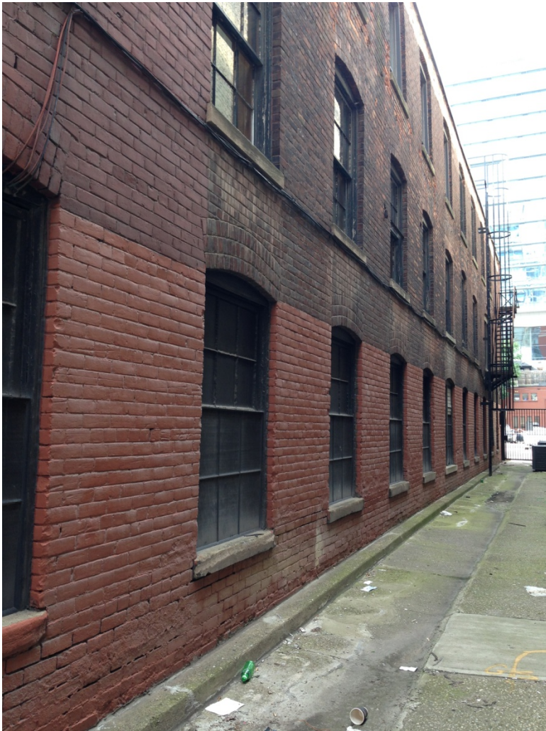
27. 352 Adelaide Street West, east (side) elevation facing former laneway (HPS,2017)
