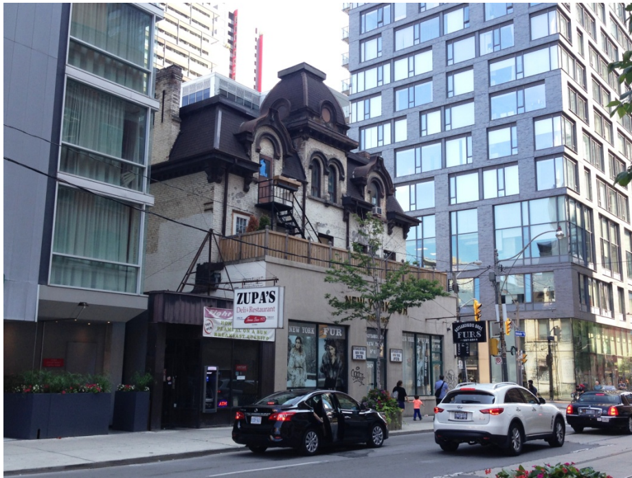
30. F + G. Perkins House, 1858, with 1876 mansard roof and 1912 storefront addition at 342 Adelaide Street West, north-west corner of Adelaide and Peter streets (HPS, 2017)
