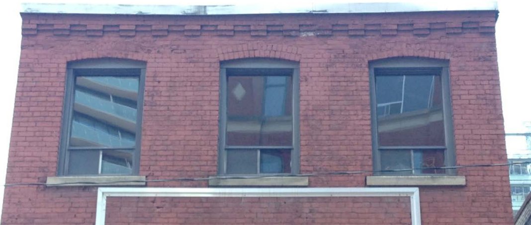
26. 352 Adelaide Street West, third floor window details and cornice (HPS, 2017)
