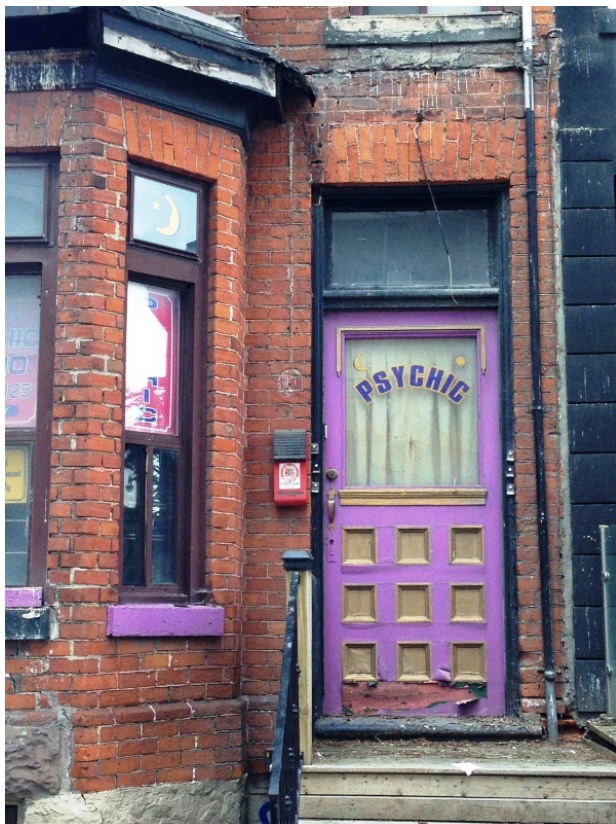
13. 118 Peter Street: showing the front door (HPS, 2017)
