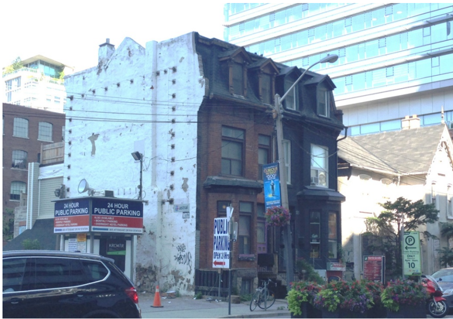
14. 118 Peter Street: showing the principal (east) and side (south) elevations. (HPS, 2017)
