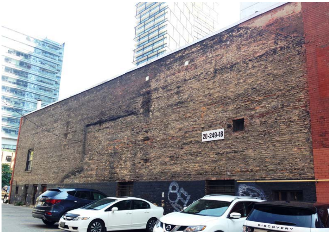
28. 352 Adelaide Street West: west (side) elevation showing the yellow brick and the 'ghost' of the previous adjacent house-form building (HPS 2017)
