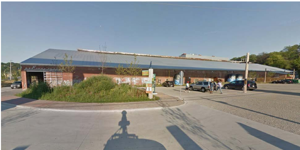
East Elevation of Building 16 (ERA Architects, Googlemaps, 2016)
