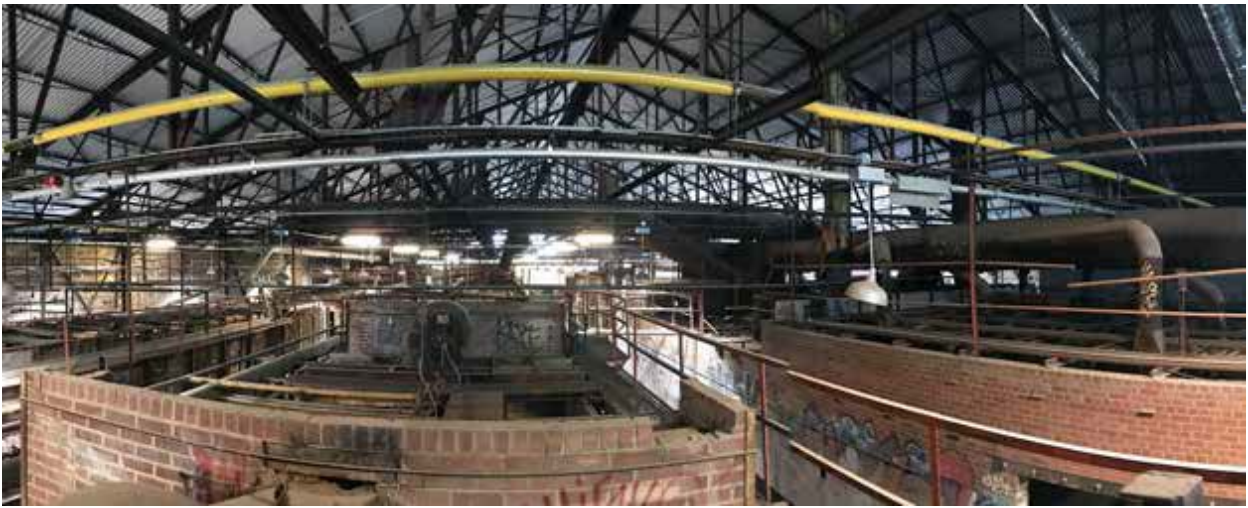
Interior of Building 16 showing the interior roof volume (ERA Architects)
