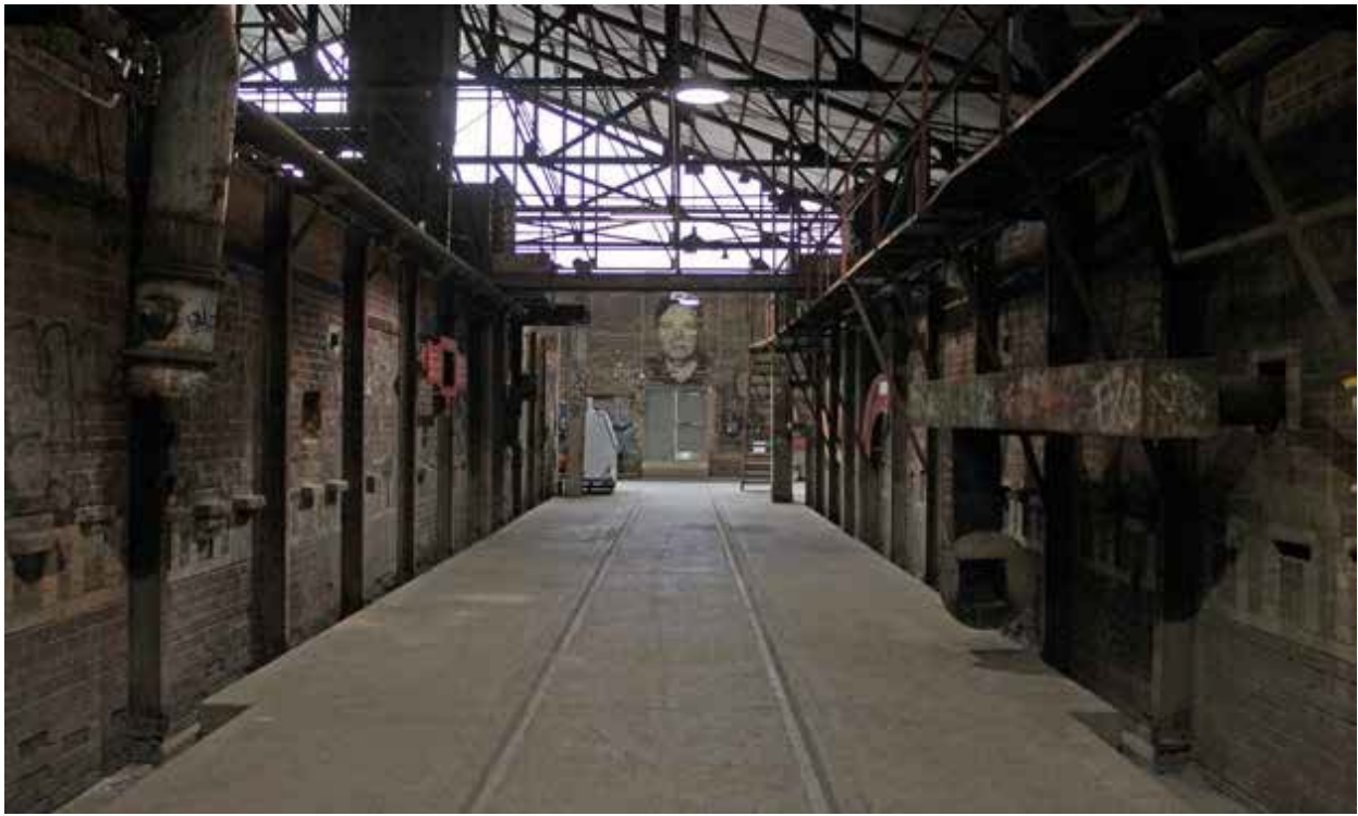
Interior of Building 16 looking north between the firing kilns (ERA Architects)
