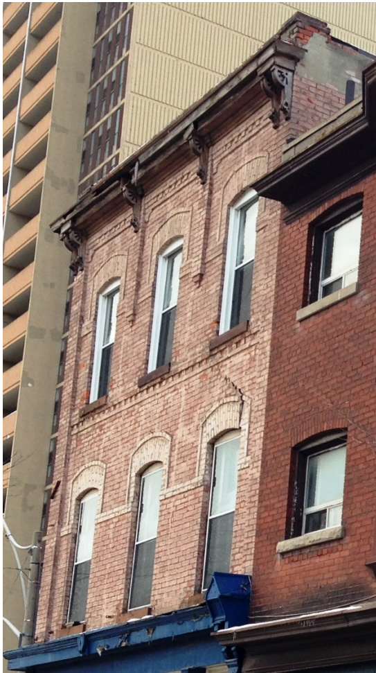
18. South Elevation: showing the details of the bricks and the cornice and brackets (HPS, 2016)
