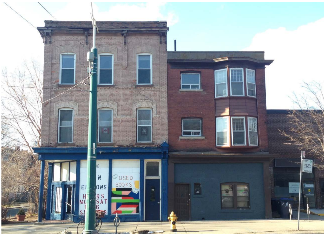
Photograph of 698 Spadina Avenue, with 700 Spadina on the right, showing the principle (east) elevations facing Spadina Avenue. (HPS, 2017)
