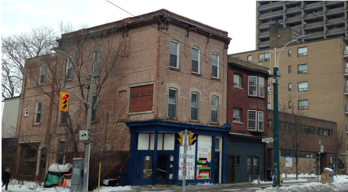
Photograph of 698 Spadina Avenue showing its principal elevation facing east towards Spadina Avenue and side elevation facing south to Sussex Avenue. To the north are 700 and 704 Spadina Avenue. (Heritage Preservation Services [HPS], 2016)
