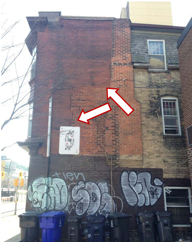
10. Photograph of the north (side) elevation of 700 Spadina Avenue showing the difference in brick and the keying of new brick with old at the left indicating the extension of the building to the east and the addition of the third storey between 1924 and 1945. (HPS, 2017)
