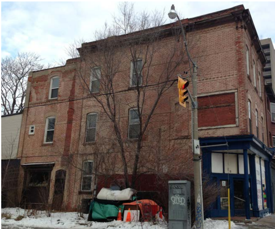
23. Side (south) elevation: showing the disposition of window openings and the side entrance and large window at the rear wing. Note the frame for a sign at the second level above the door also evident in Image 13 and 17 etc. (HPS, 2016)
