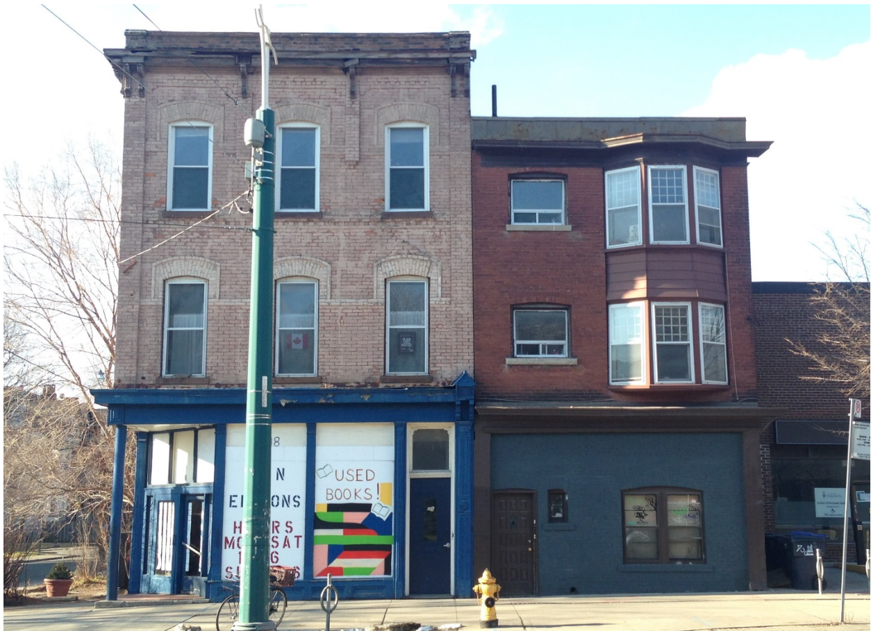
14. 698 and 700 Spadina Avenue: showing the principal (east) elevation (HPS, 2017)
