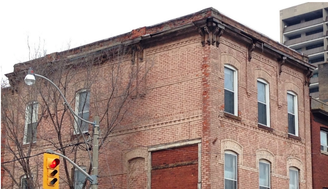
17. South and east elevations: showing the decorative brick banding, buff brick window headers, pilasters, drop pendants of the upper two floors. (HPS, 2016)
