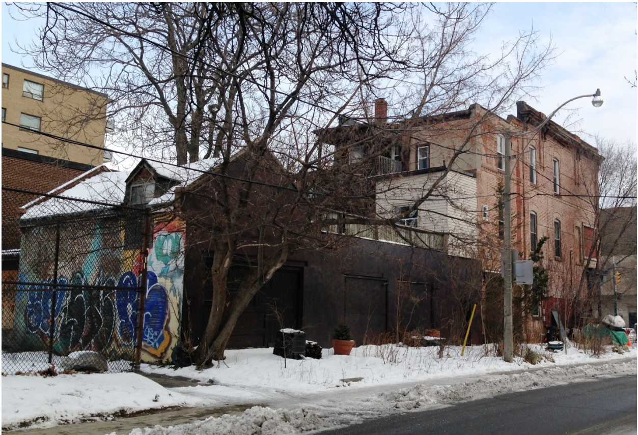
16. 698 Spadina Avenue, side (south) elevation: showing the rear view of the property and the gable-roofed outbuilding with its dormer windows and the walls enclosing the property. (HPS, 2016)
