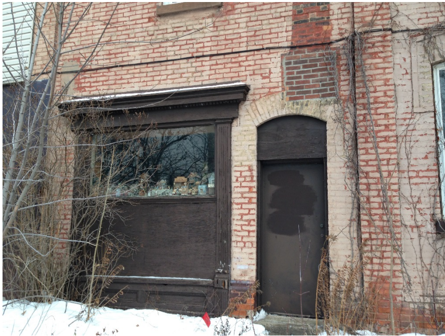
24. Side (south) elevation: showing the side entrance and large window with decorative wood framing. (HPS 2016)
