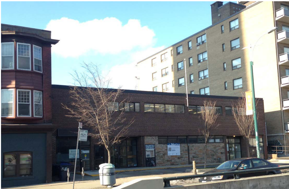
Photograph of 704 Spadina Avenue, showing the principle (east) elevation facing Spadina Avenue. (HPS, 2017)
