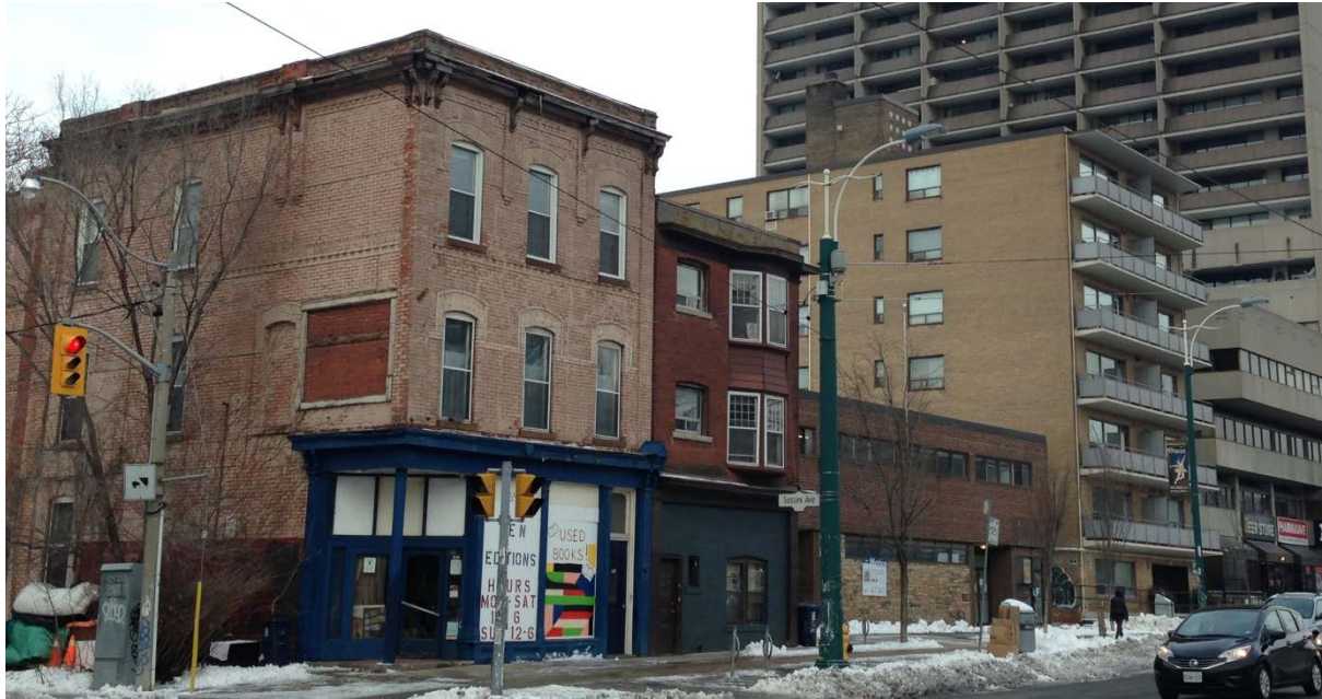
13. Photograph of the north-west corner of Spadina and Sussex avenues with the original building at 698 Spadina Avenue, the extended and altered building at 700 Spadina Avenue and the two-storey block at 704 Spadina Avenue dating from 1972 (HPS, 2016)
