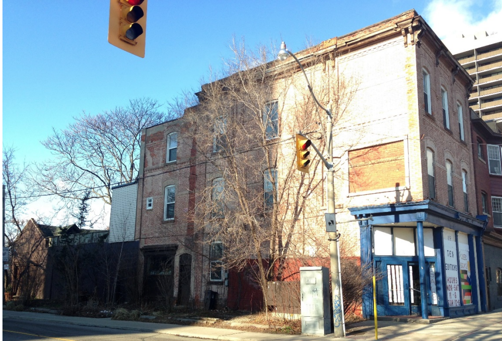
15. 698 Spadina Avenue showing the side (south elevation) with the lower rear wing, clapboard sunroom (1945) and the one-storey wall enclosing the property and linking with the rear gable roofed out building. (HPS, 2017)
