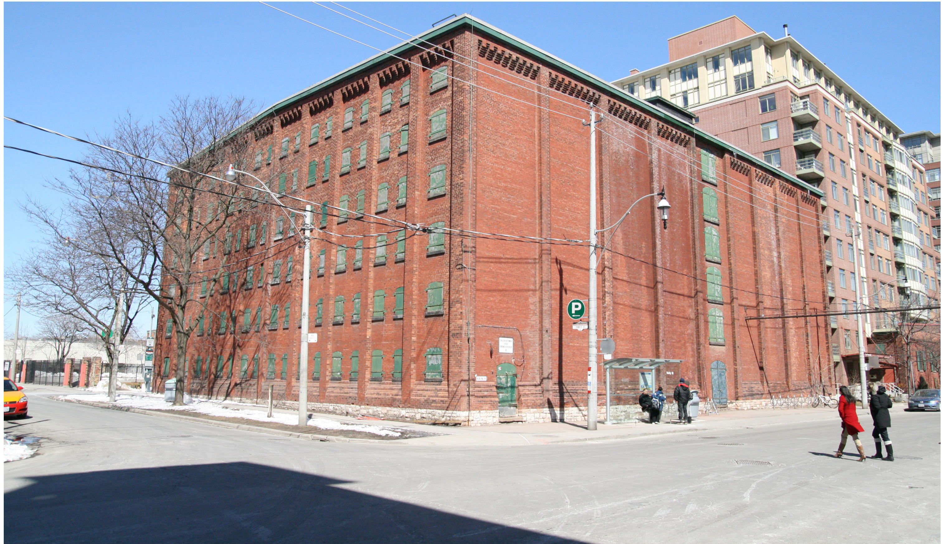
Rack House D | 60 Mill Street
