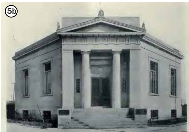
IMAGE 5. 1921 Bank of Montreal (Construction, p. 371)
