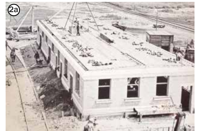
IMAGE 7. 1916 August 24 Harbour Commission building under construction (Toronto Harbour, The Passing Years)
