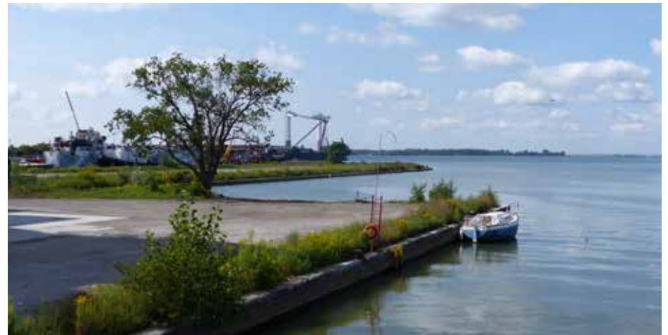
IMAGE 4. Cousins Quay, existing conditions
