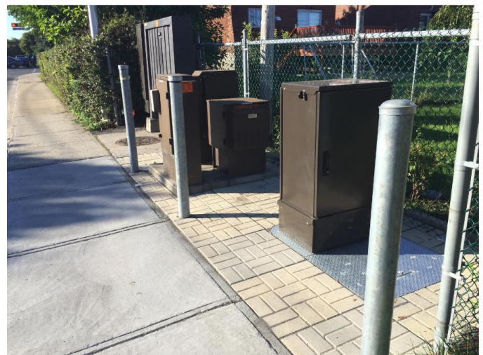
Clustering of equipment – no aesthetic treatment
