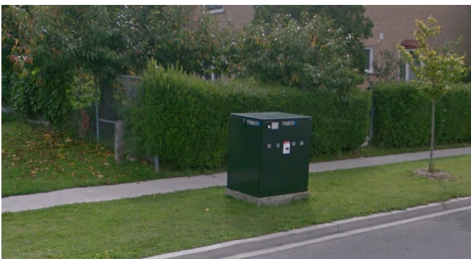
Tap box placed behind fence/hedges at the flank of a house
