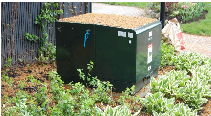
Equipment placed next to a driveway behind a fence. Picture credit: Toronto Hydro
