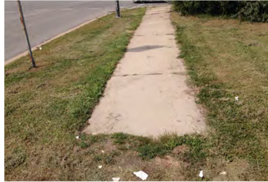
Lack of connections throughout the Centre
