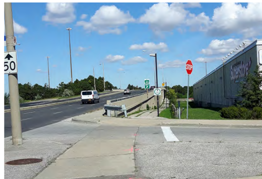
Highway 401 is a barrier to pedestrians and cyclists
