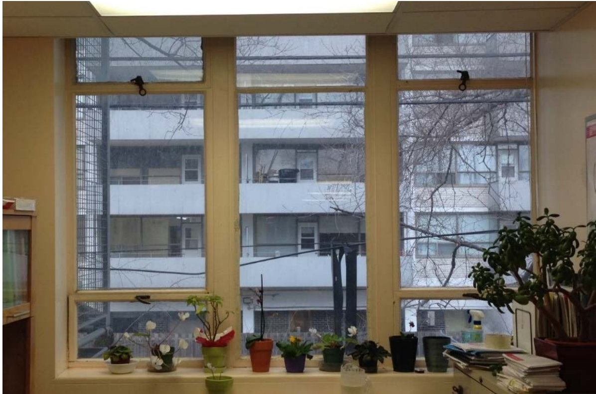
31. Interior view of typical steel section windows in the second floor north office (below) with brass openers (HPS, 2017)
