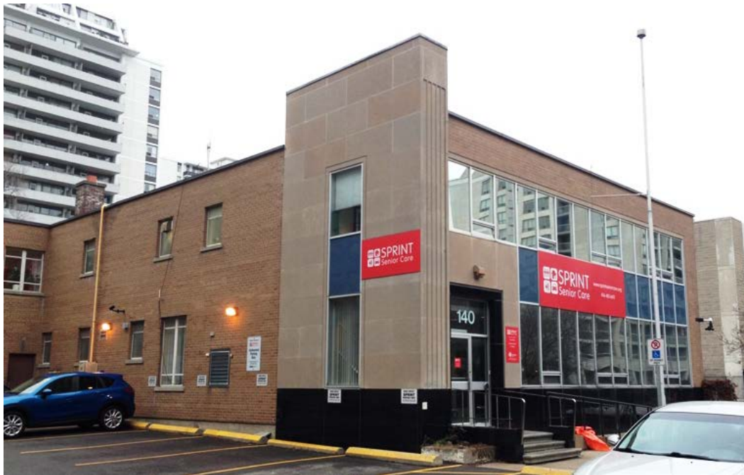
29. Side (west) and principal (south) elevations: showing the west elevation with its steel windows for a ground floor office and washrooms (smaller). The ground floor window, and that viewed in the upper corner represent typical glazing system of the east, west and north elevations with opening systems at the top and bottom of the window to provide a variety of options to enhance comfort and cross ventilation. (HPS, 2017)
