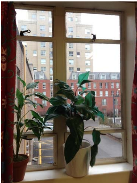
30. Interior view of typical steel section windows in the west staircase (above) with brass openers (HPS, 2017)
