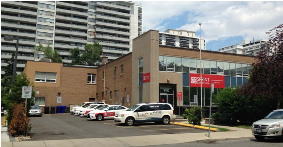
12. 140 Merton Street: photograph showing the principal (south) elevation and the west side of the property. At the rear of the property, the 1985 infill addition at the second floor level can be detected with the different coloured brick (HPS, 2016)
