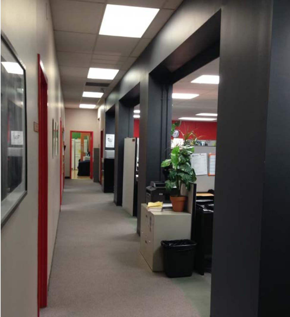
21. Interior on the east side of the second floor showing the original external wall (at the right) of the narrower upper floor prior to the extension (centre and left) in 1985. (HPS, 2017)
