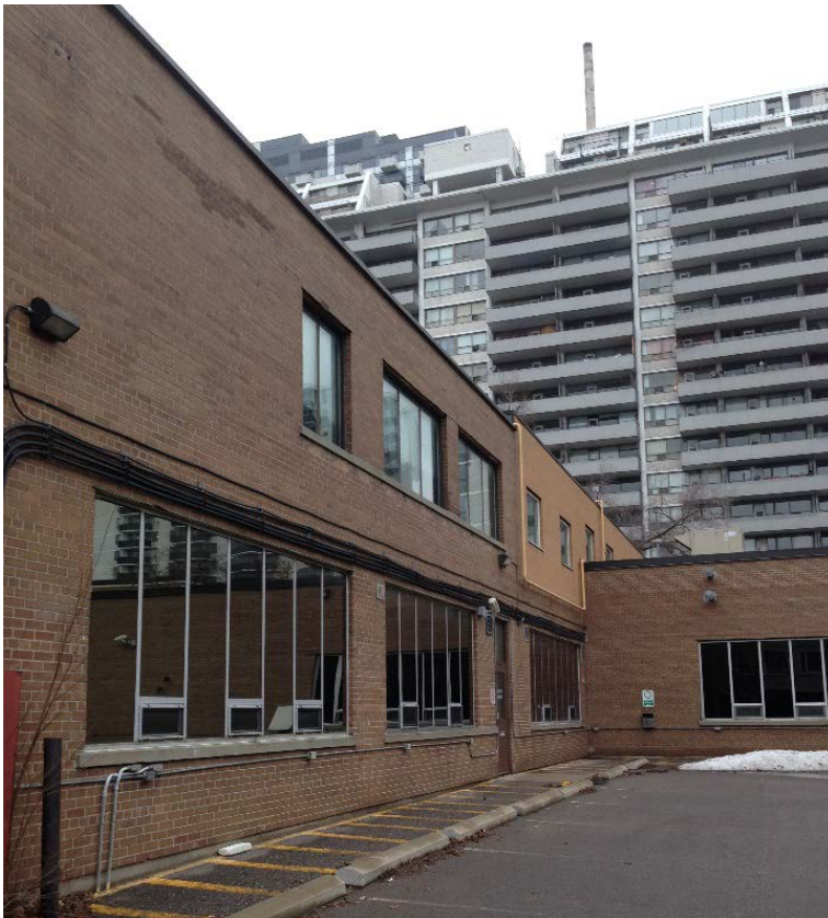
28. East elevation showing the office windows (left). The ground floor windows were likely replaced in 1973 as they match those of the warehouse extension (to the right). The pattern of mullions and lower opening sections corresponds to the front, south elevation, curtain wall. The windows at both levels, while maintaining the original pattern are new glazing systems (HPS, 2017)
