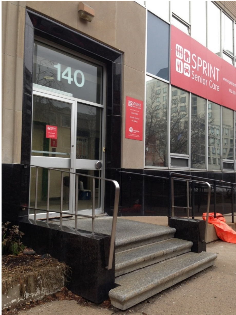
23. Entry at 140 Merton Street, viewed from the west: showing the granite steps flanked by polished black granite base for the balustrade and the door frame with later ramp handrails to the right in black hollow metal tubing and the curtain wall details with the opening sections (HPS, 2017)
