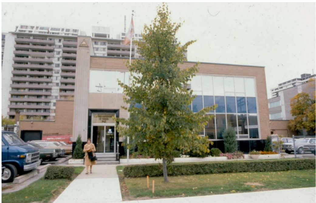
11. 140 Merton Street: photograph taken between 1973 and 1985 showing the 1973 addition on the right at the rear of the property. On the left side of the photo, the 1985 second storey addition has not yet been added, nor the delivery access door removed. The parking in front of the building has been replaced by a landscaped open space (War Amps Archives, Scarborough)
