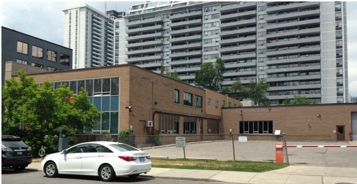
13. 140 Merton Street: photograph showing the principal (south) elevation and the east side of the property. Note at the rear of the original building, the second-storey addition constructed in 1985 indicated by the different coloured brick, as well as the single-storey addition, at the rear of the parking lot completed in 1973. (HPS, 2016)
