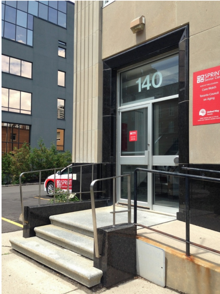
24. Entry at 140 Merton Street, as seen from the east: showing the details of the entrance and the fluted pier with the later ramp and handrail to the right of the step (HPS, 2016)
