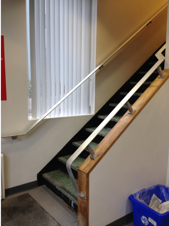
33. Entry Stairs in lobby adjacent to elevator showing: green terrazzo treads and balustrade trimmed in wood with a handrail similar to the exterior stairs (HPS, 2017)
