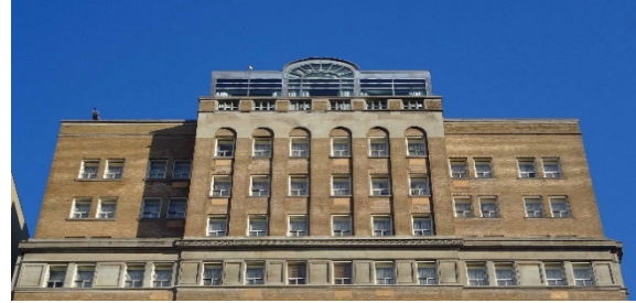
4e. south roofline detailing
