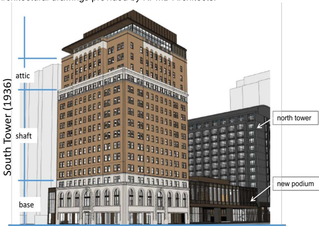
View of the south tower showing the new three-storey retail addition to the west and new podium link to the north tower (right side of image)
